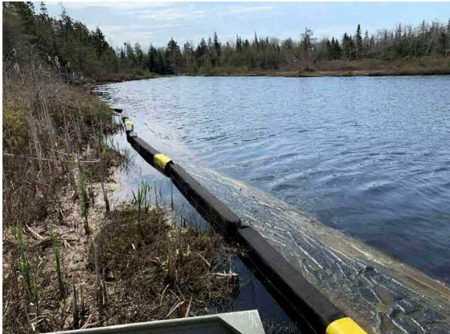
Photo 2: Silt Boom in Sheas Lake
