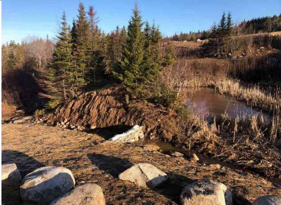
Photo 1: Sand bag berm placed in the ditch North West side of the Turn around..
