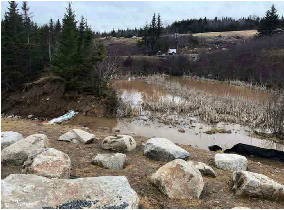
Photo 3: Water accumulated behind berm, Water being pumped through filter bags from this location.
