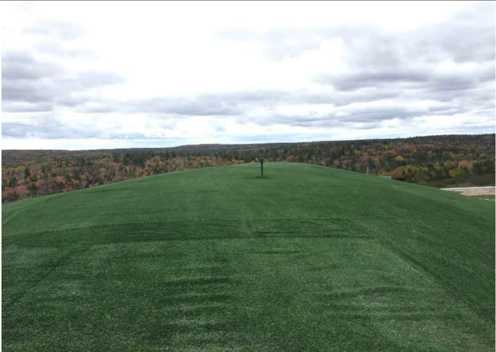
Photo 18: Western view of the top of the main landfill cell area (capped) - eastern portion of cell.
