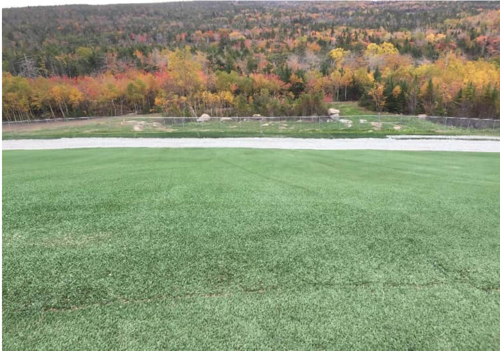
Photo 23: Southern view taken from the middle top area of the main landfill cell area (capped).
