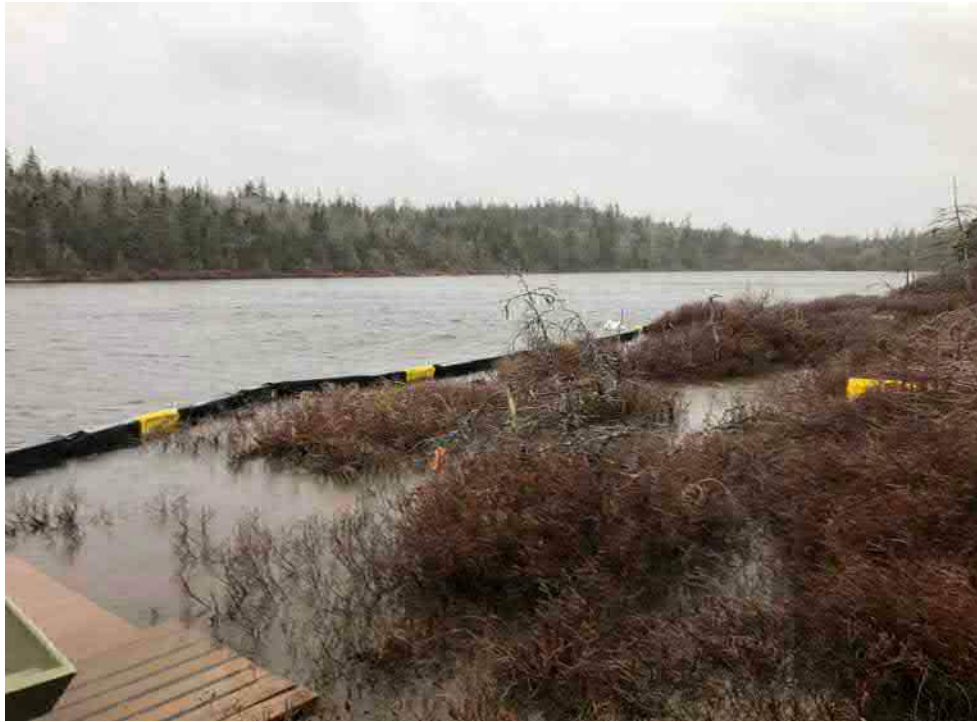
Photo 3: Silt boom installed in Sheas Lake (10:10am).
