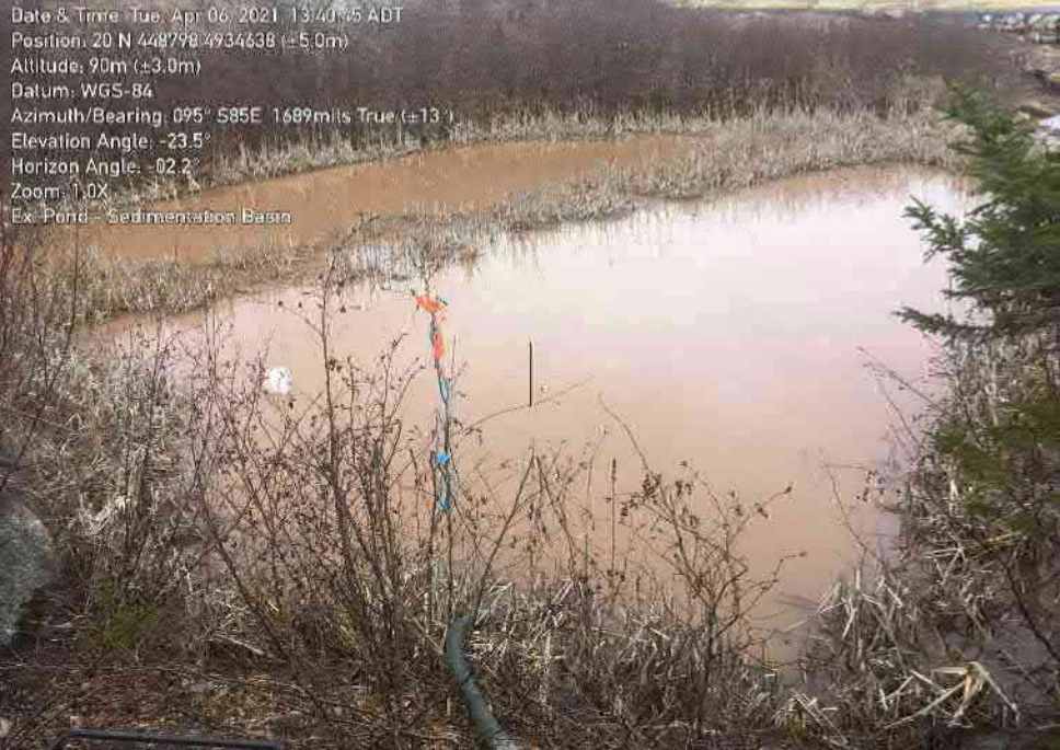
Photo 11: Existing pond with suspended sediment - pumped and filtered through silt sack - continual monitoring and pumping/filtering as required.
