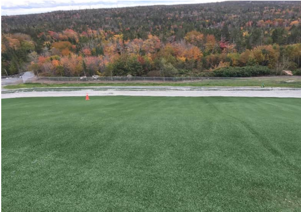
Photo 21: Southern view taken from the eastern top area of the main landfill cell area (capped).
