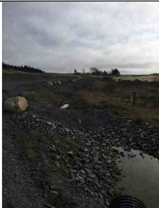
Photo 2: Check dam in the ditch north of the landfill cell.
