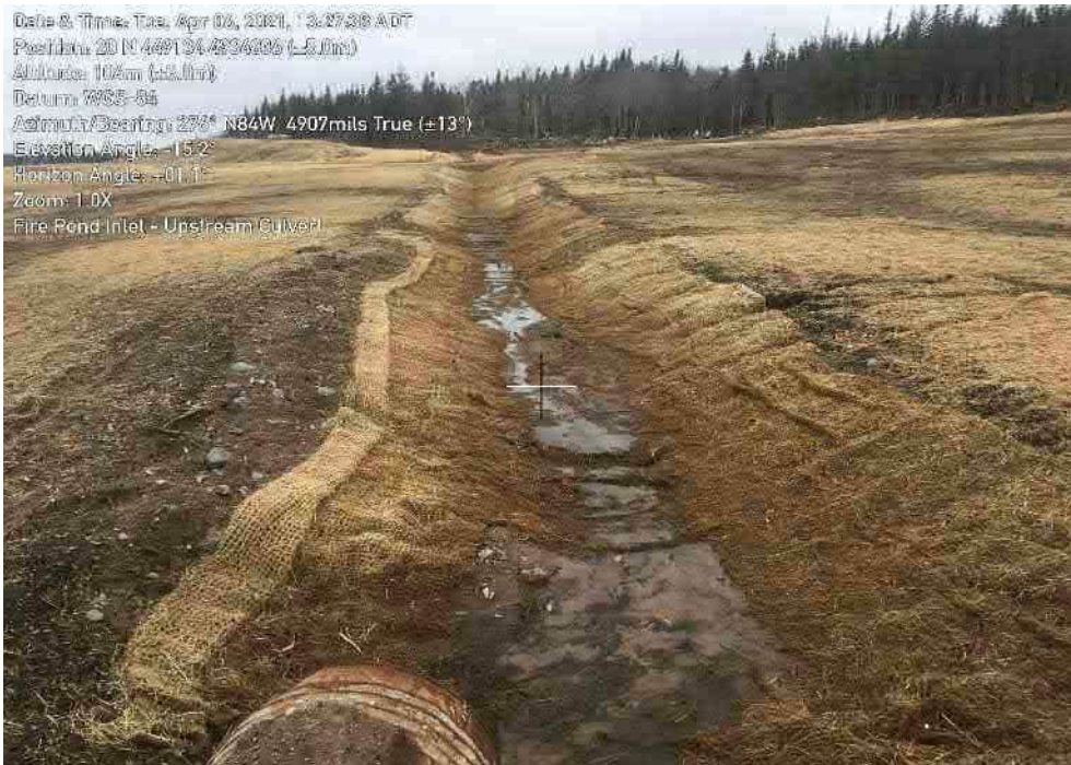
Photo 4: Channel upstream of existing damaged culvert. Good condition.
