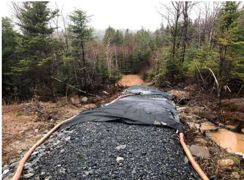
Photo 4: Water pumped through filter bags.
