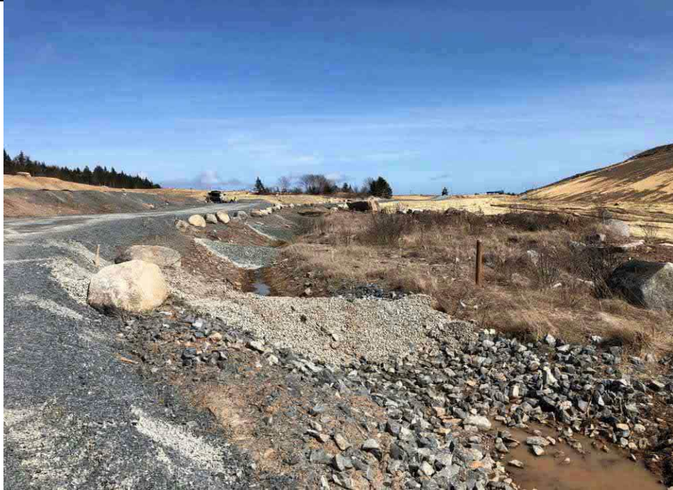
Photo 3: Check dam installation..
