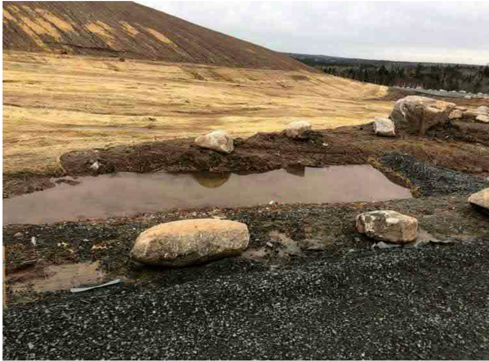
Photo 1: Water accumulated behind check dams.
