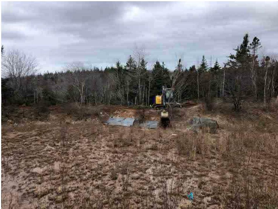
Photo 4: Repairs to the settling pond west of the turnaround area.
