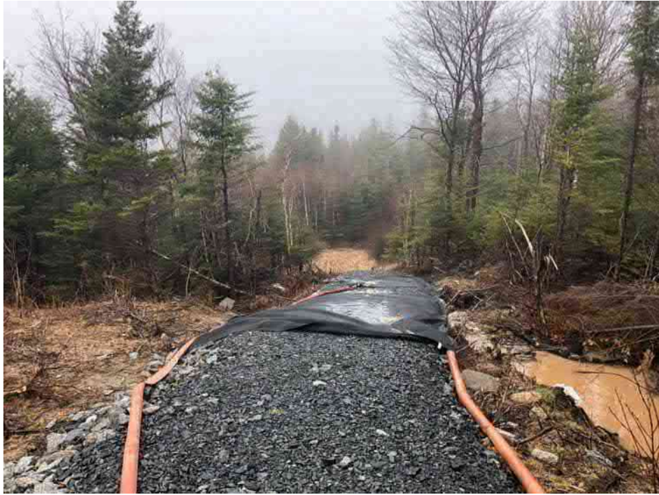
Photo 7: Pumping silty water, using filter bags to reduce silt.
