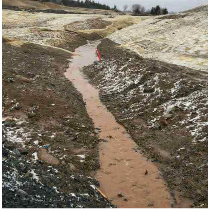
Photo 5: Ditch north of landfill cell (3:40pm).
