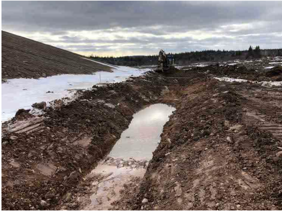
Photo 5: ARCP continues digging lined trench. Some bedrock encountered.
