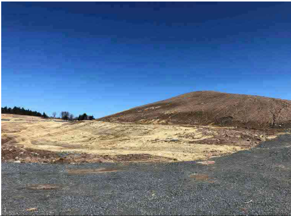
Photo 1: Landfill cell looking East.
