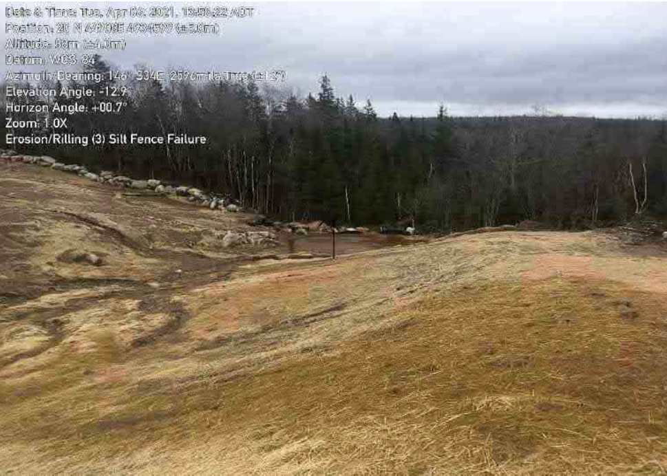
Photo 21: Southeast corner of landfill cap slope. Heavy erosion occurring. Re-grading and slope stabilization required, additional erosion control matting and biofilter check dams in localized channel. Silt fence failure and accumulated
