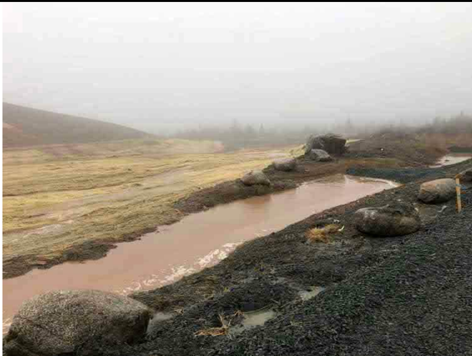
Photo 6: Check dam in the ditch north of the landfill cell.
