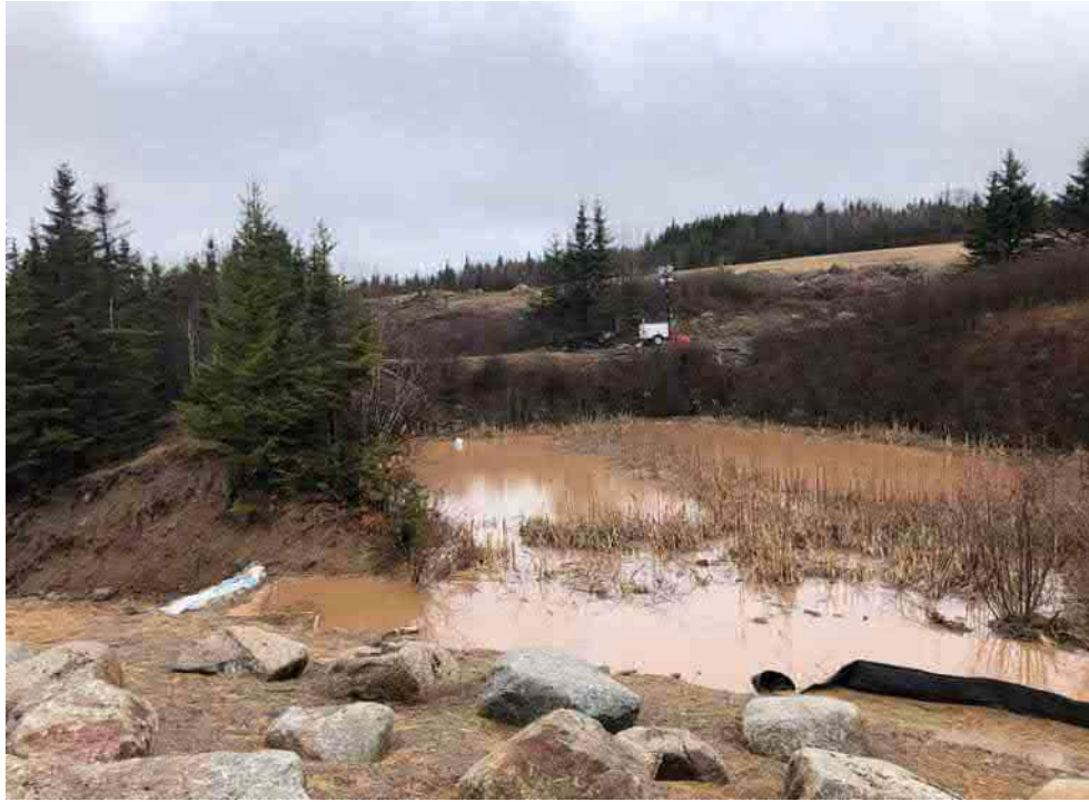
Photo 5: Silty water being pumped into filter bags.
