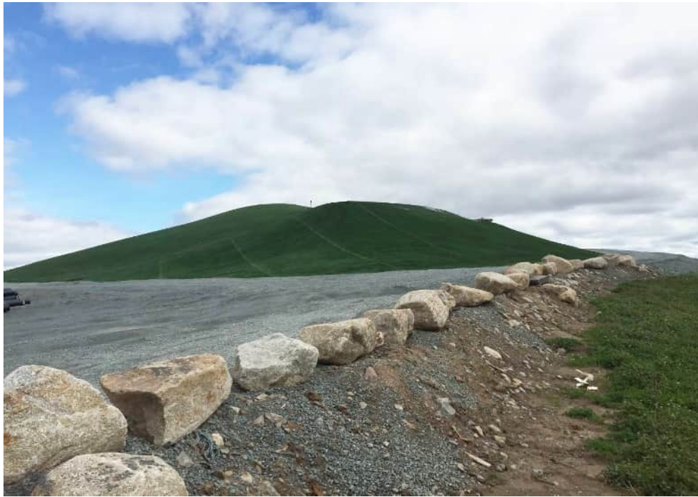
Photo 13: Eastern view of the western of the main landfill cell area (capped)
