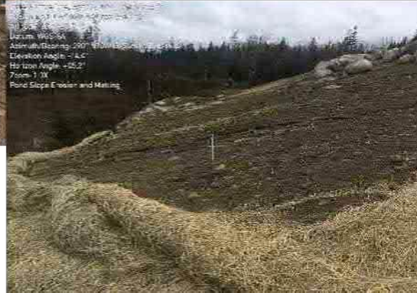
Photo 15: Slope exposed and unprotected/stabilized. Heavy erosion occurring. Rolled erosion control products required to stabilize slope. Failure to secure erosion matting.
