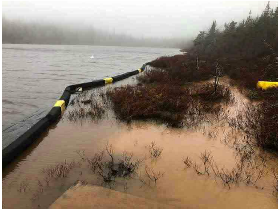
Photo 8: Silt control along the shoreline west of BDA I.
