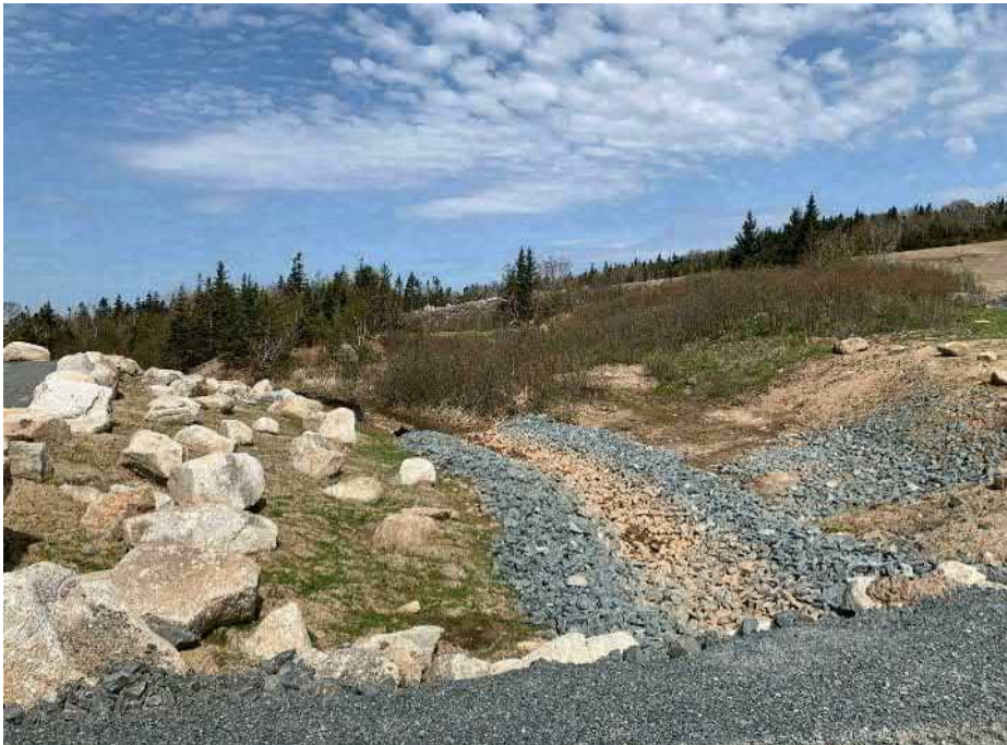
Photo 6: Rocks placed in ditch by turnaround pad.
