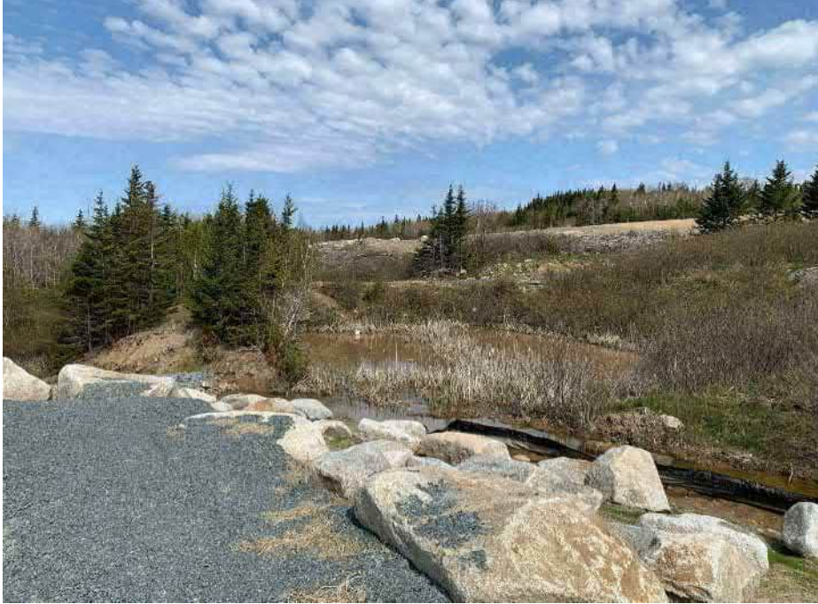
Photo 5: Hay bail and rock dam holding water North of the turnaround pad.
