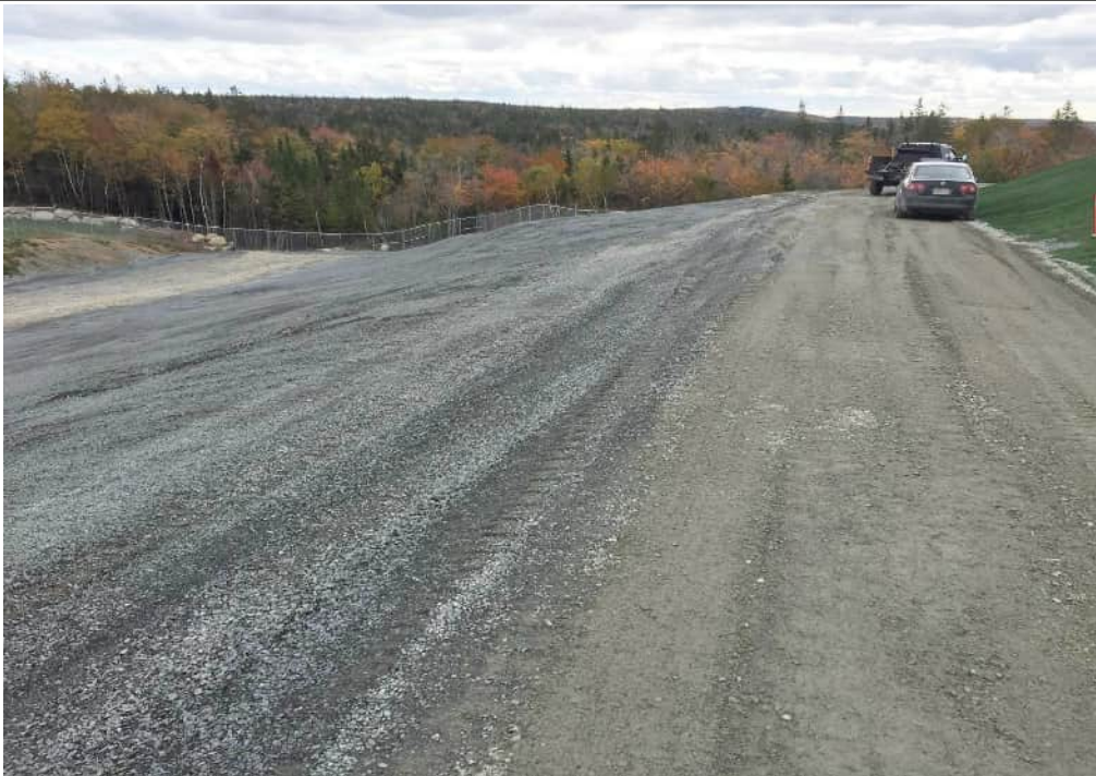
Photo 6: Southern view of the eastern slope area (capped).
