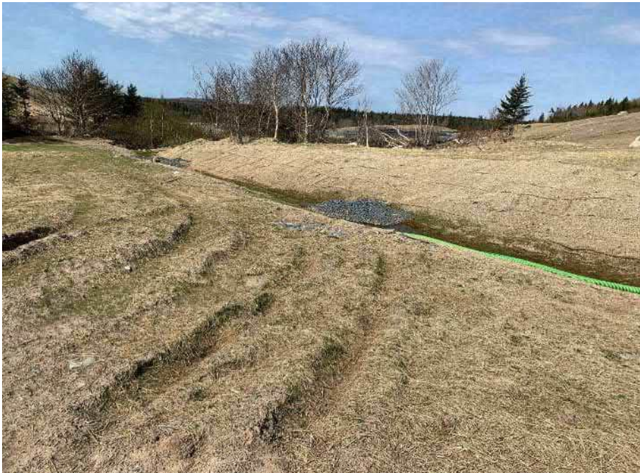
Photo 12: Cocomatting, hay bail and rock check dams placed in ditch dug through former BDA CDELM. The ditch travels from the North of the site to the access roadway ditching.
