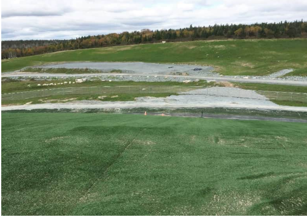
Photo 17: Northern view taken from the middle top area of the main landfill cell area (capped).
