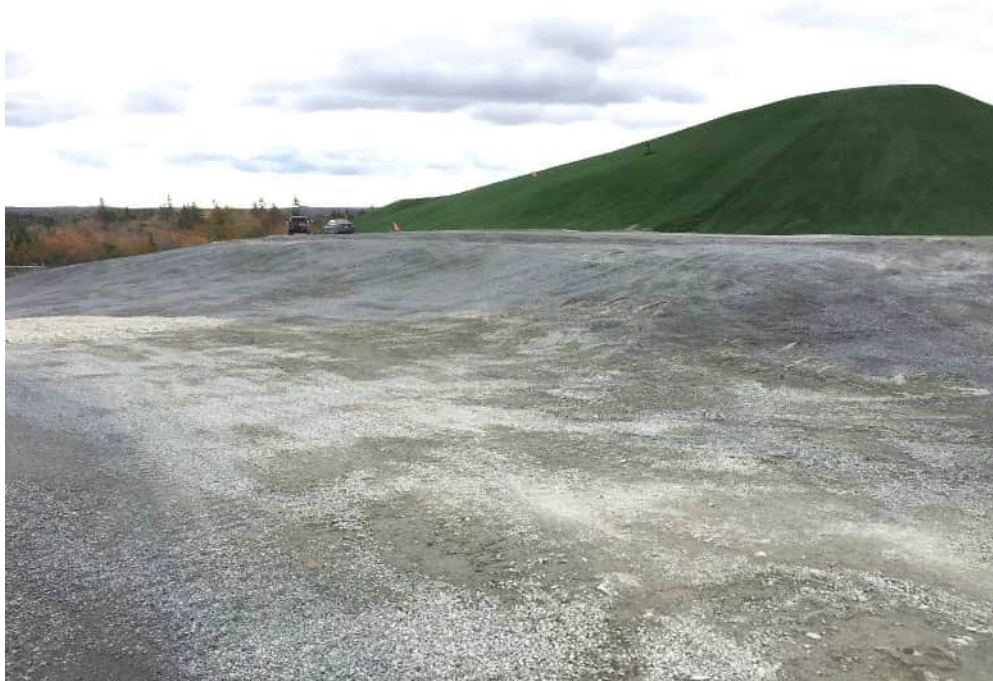
Photo 4: Southwestern view of the eastern slope area (capped).
