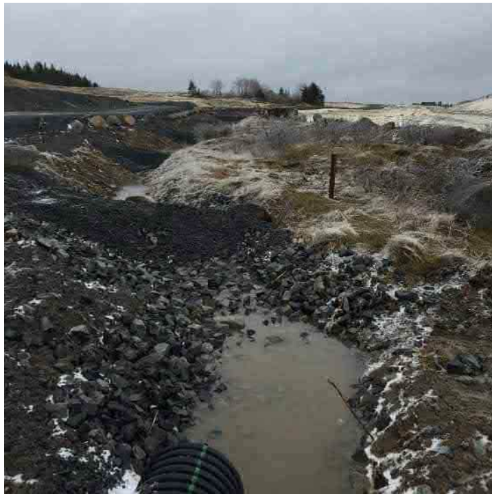
Photo 4: Check dams along access road (3:35pm)
