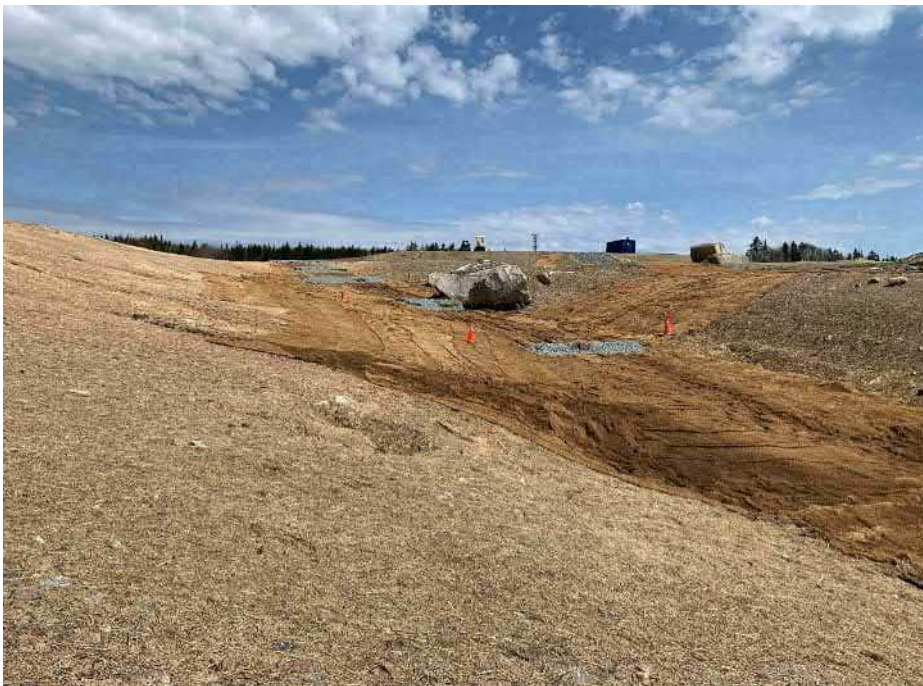
Photo 4: Looking from the basin up towards the asphalt pad. Cocomats and hay bails covered in gravel down the middle of the swale.
