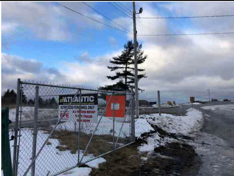
Photo 2: Asbestos signage from previous demolition work. Signage was removed.
