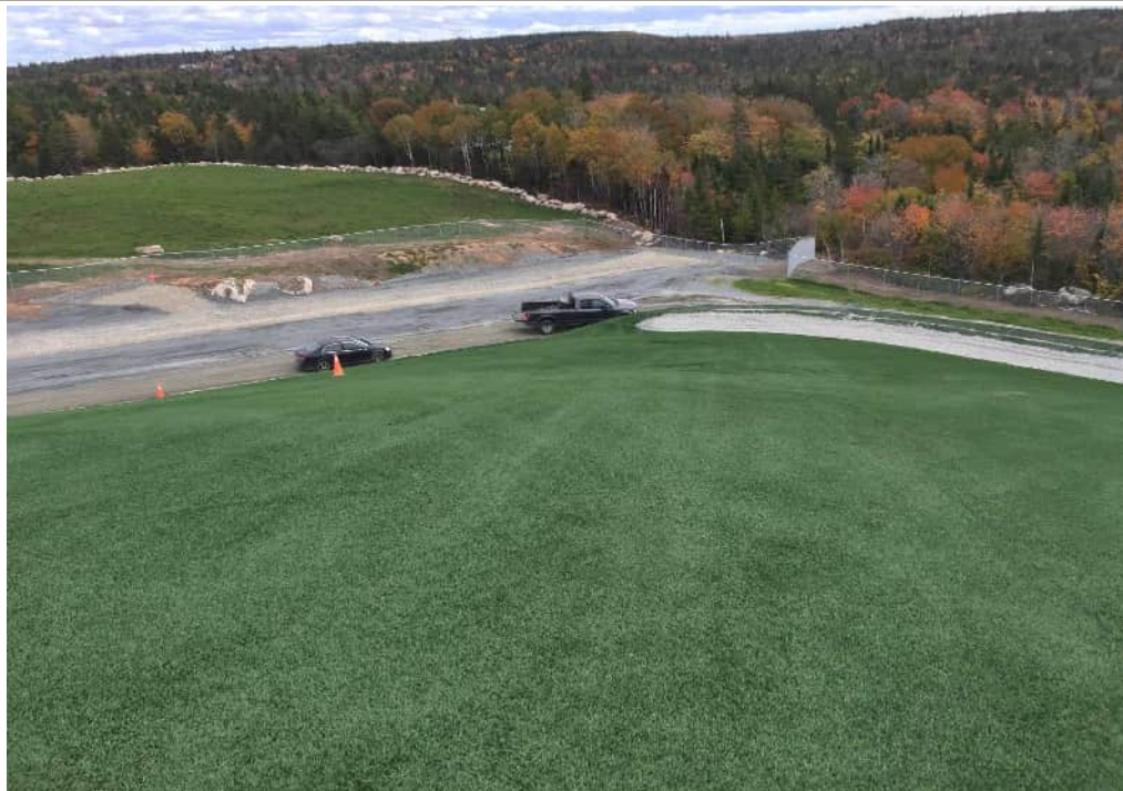
Photo 20: Southeastern view taken from the eastern top area of the main landfill cell area (capped).
