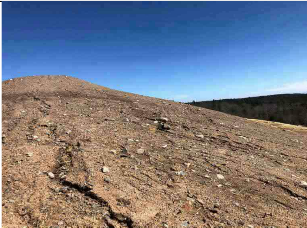
Photo 2: Rocks exposed in the landfill cap.
