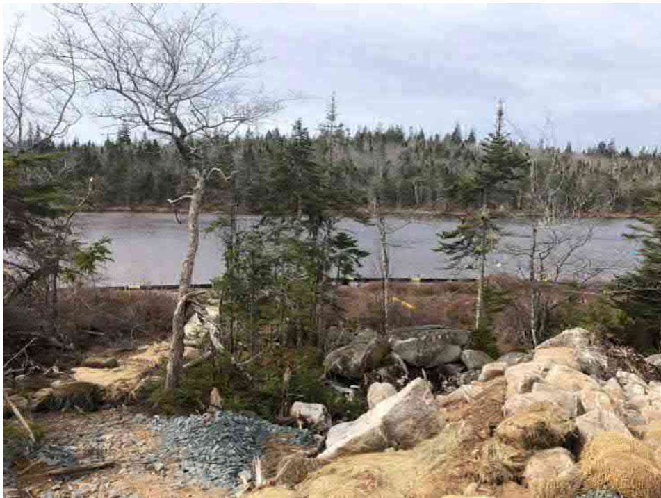
Photo 2: Silt boom installed in Sheas Lake.
