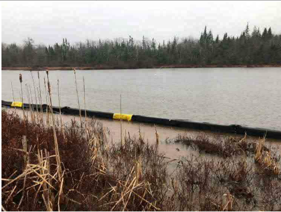
Photo 5: Silt boom providing silt control within Sheas Lake.
