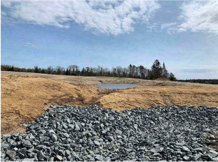
Photo 13: Cocomatting, and rock lined ditch for outflow of old fire pond.
