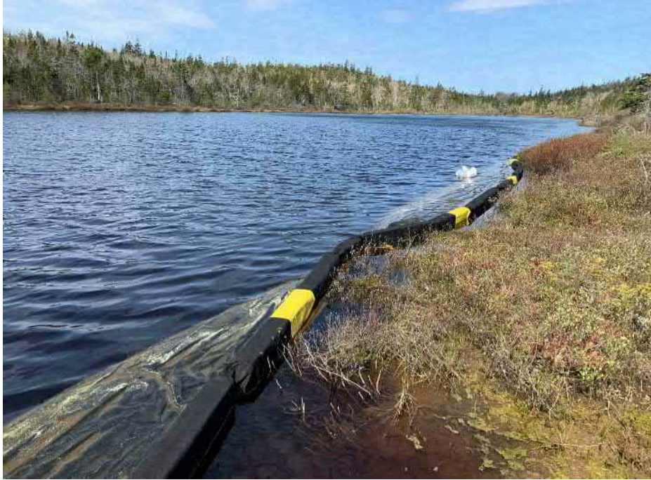
Photo 1: Silt Boom in Sheas Lake.
