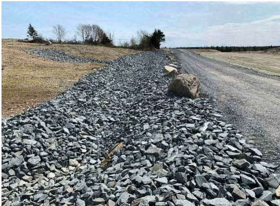
Photo 10: Rock lined ditch along the North side of the access roadway.
