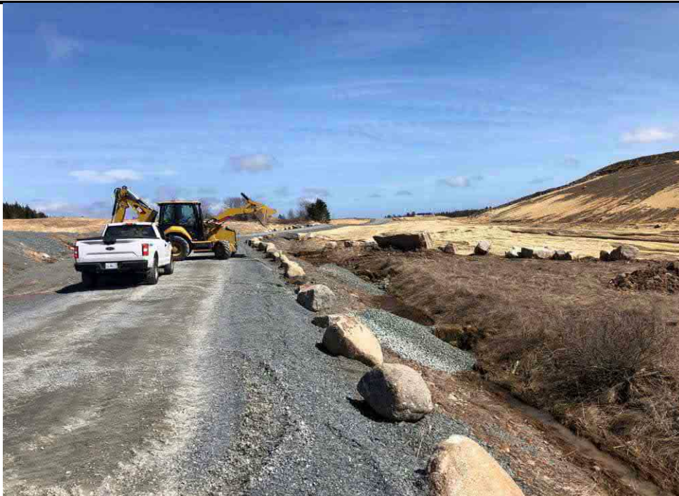
Photo 2: Check dam installation.
