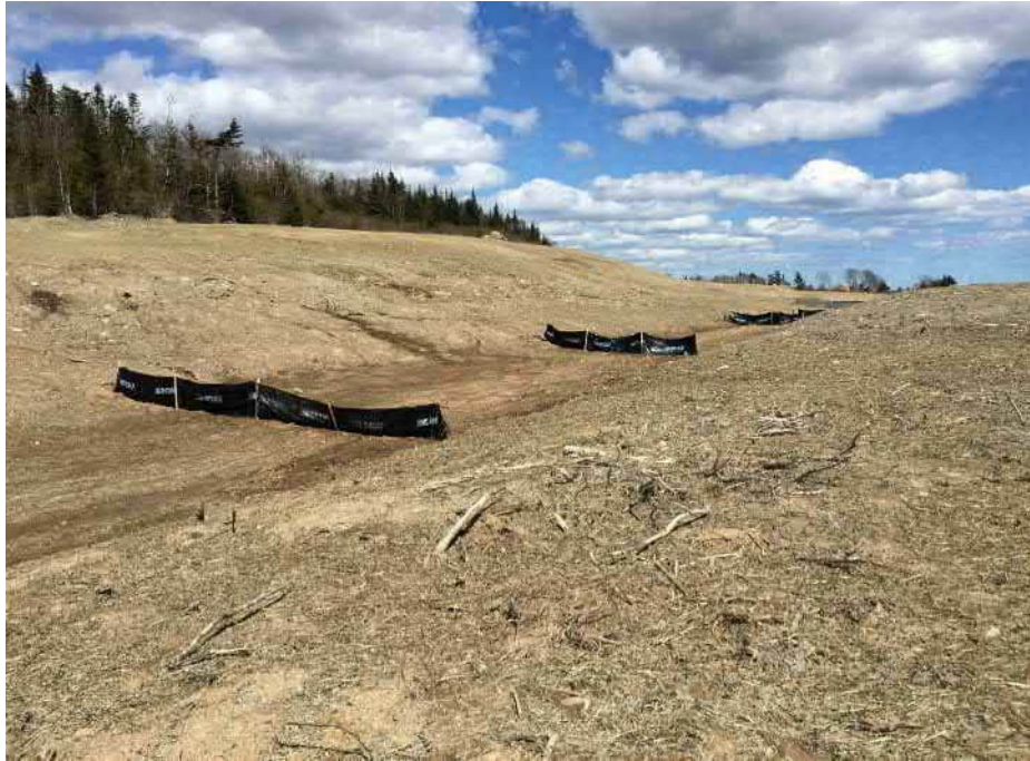
Photo 15: Silt fencing in swale of the old borrow area.
