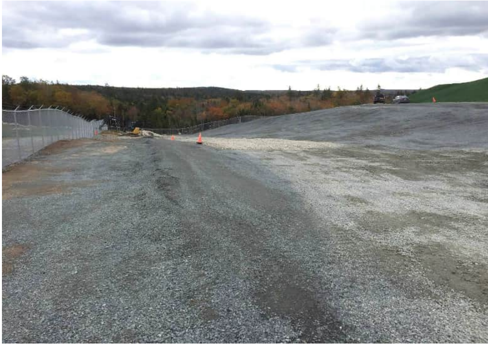
Photo 5: Southern view of the eastern slope area (capped).
