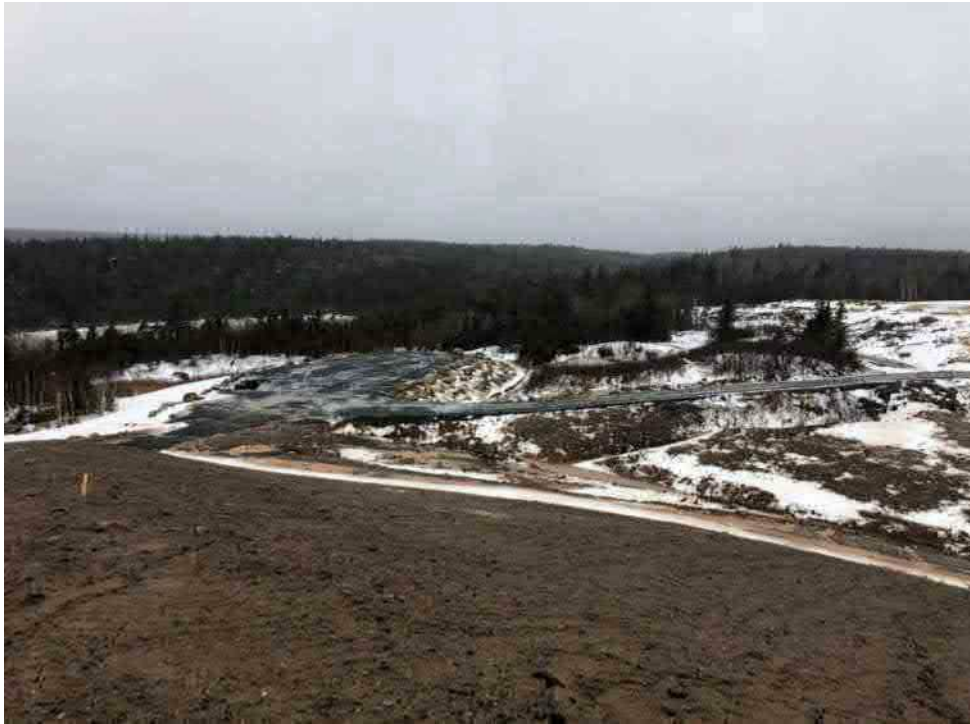
Photo 1: Some silty water in the newly constructed lined ditch, 3 check dams in place to help manage silt.
