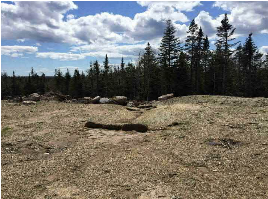
Photo 14: Hay blankets and bails placed in swale to the northwest of the old borrow area.
