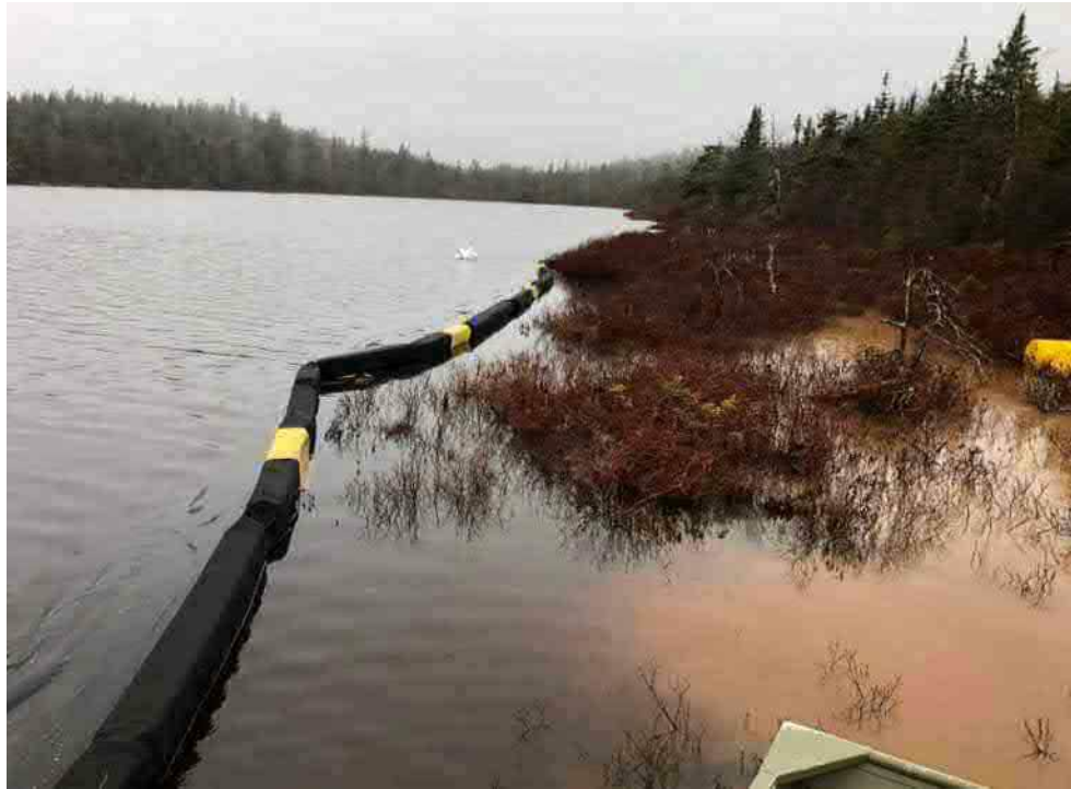
Photo 3: Silt containment along the edge of Sheas Lake.
