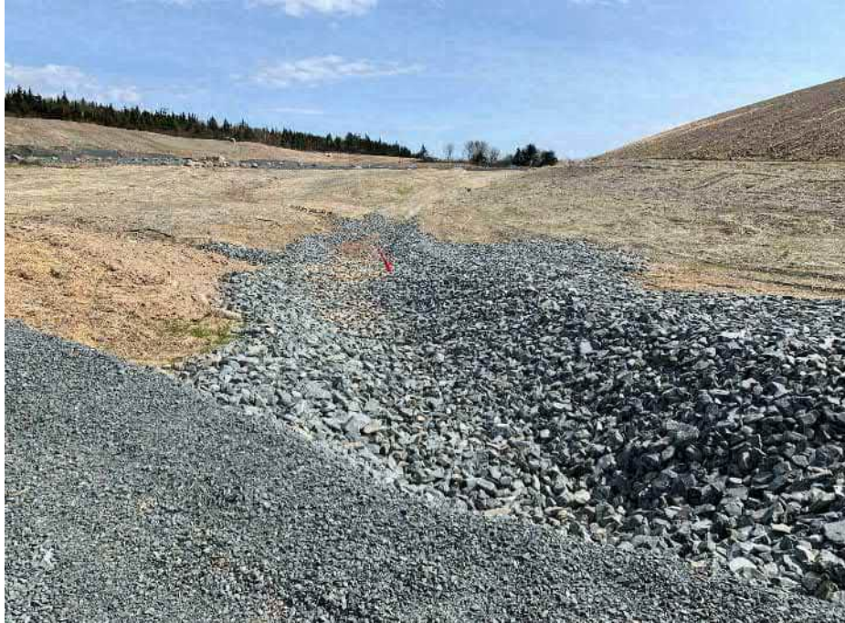
Photo 7: Rock lined ditches North of the landfill cell.
