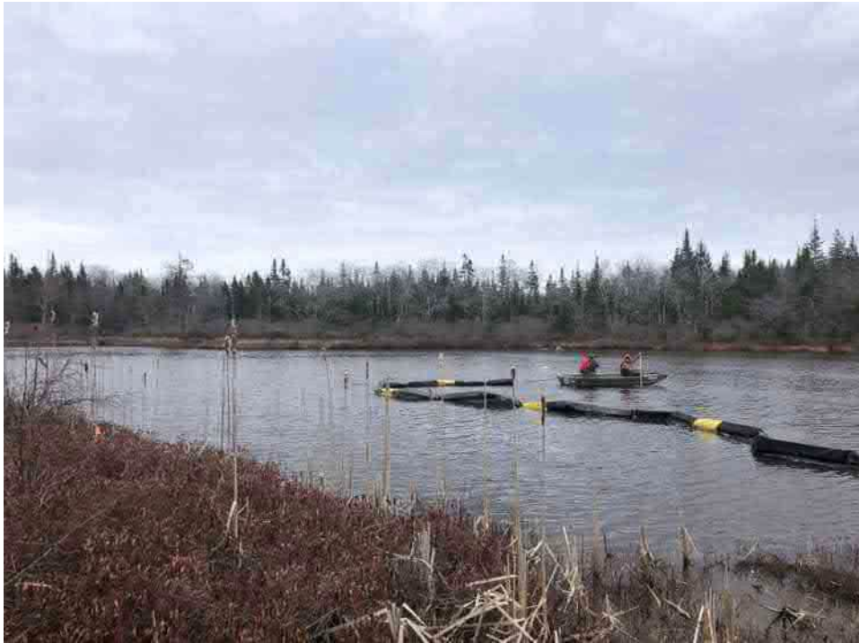
Photo 1: Silt boom being installed in Sheas Lake.
