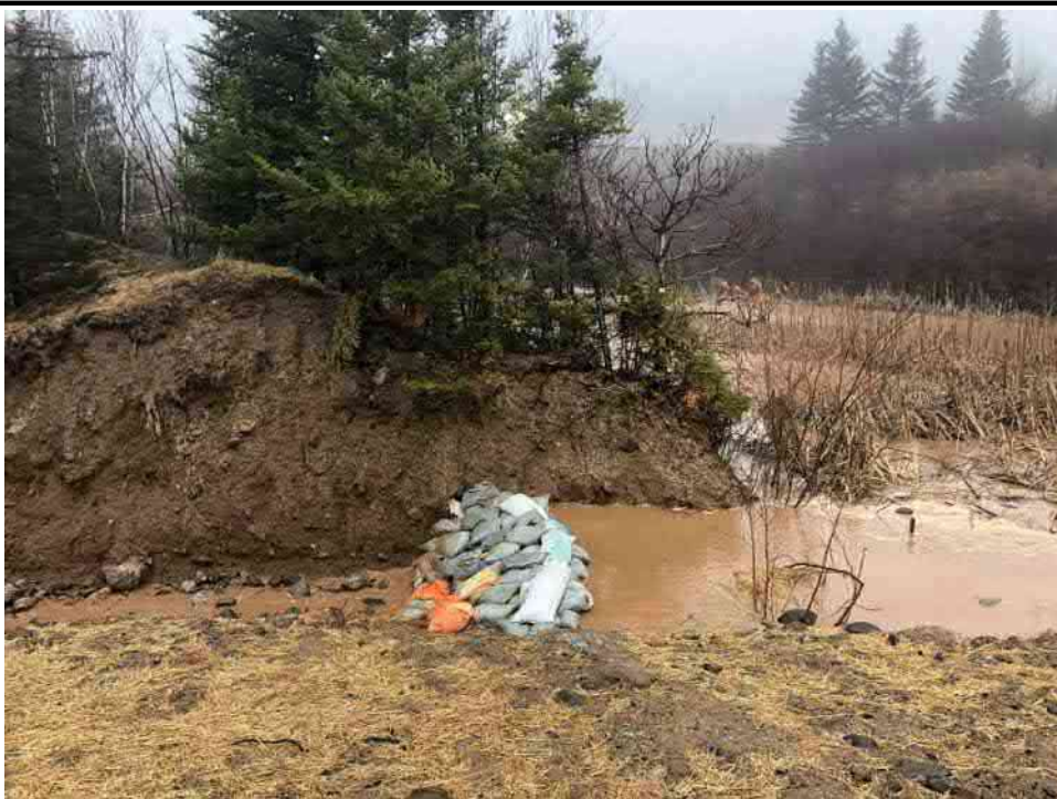
Photo 9: Berm northwest of turn around area to reduce surface water flow.
