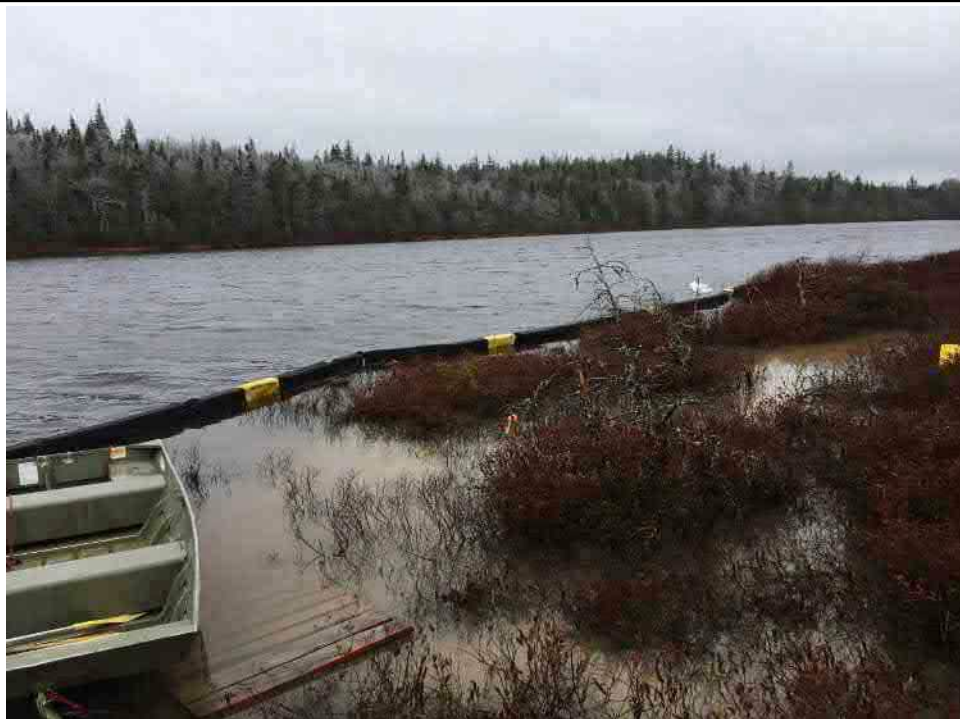
Photo 8: Silt control boom area along the shoreline west of BDA I (3:55pm).
