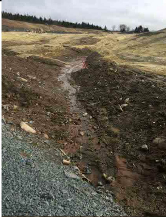
Photo 3: Drainage ditch on north side of landfill cell
