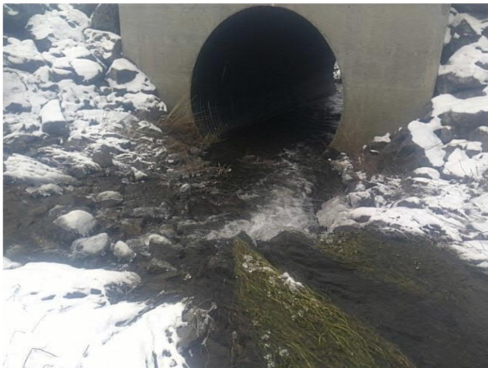
Photo No. 11: View of COB-4-SW looking west.
