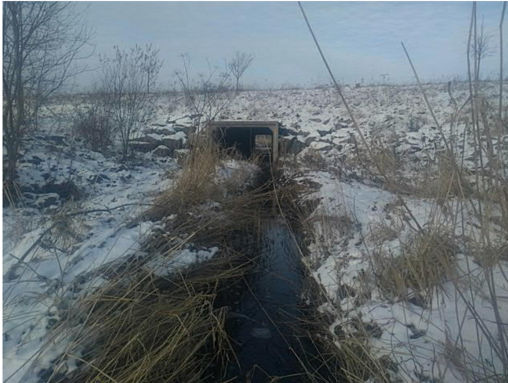
Photo No. 1: View of CB-SW looking northwest.
