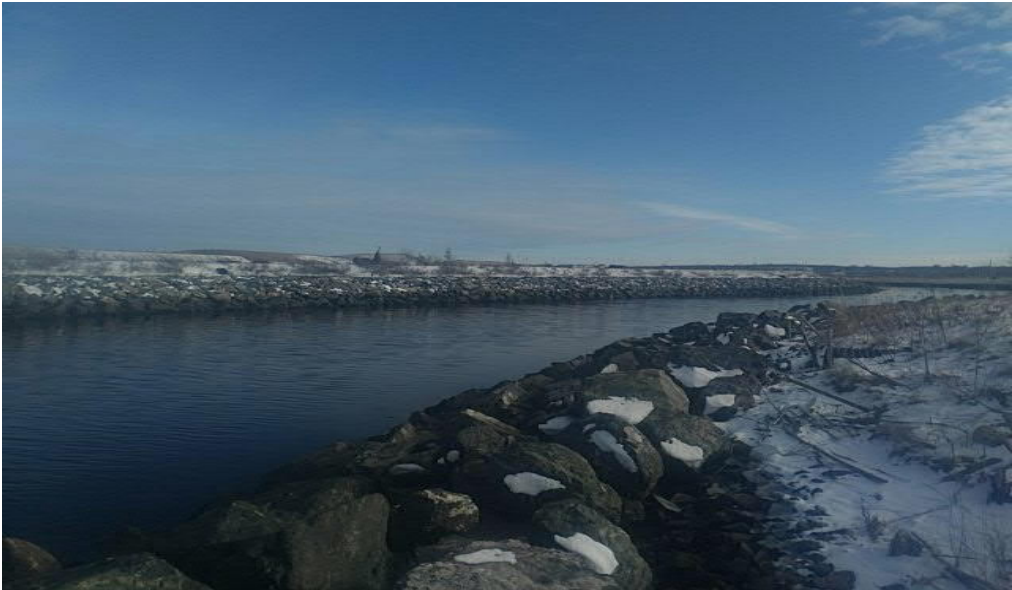
Photo No. 20: View of BP-1-SW looking east.
