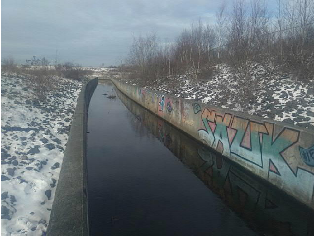
Photo No. 5: View of SRC-1-SW looking northwest.
