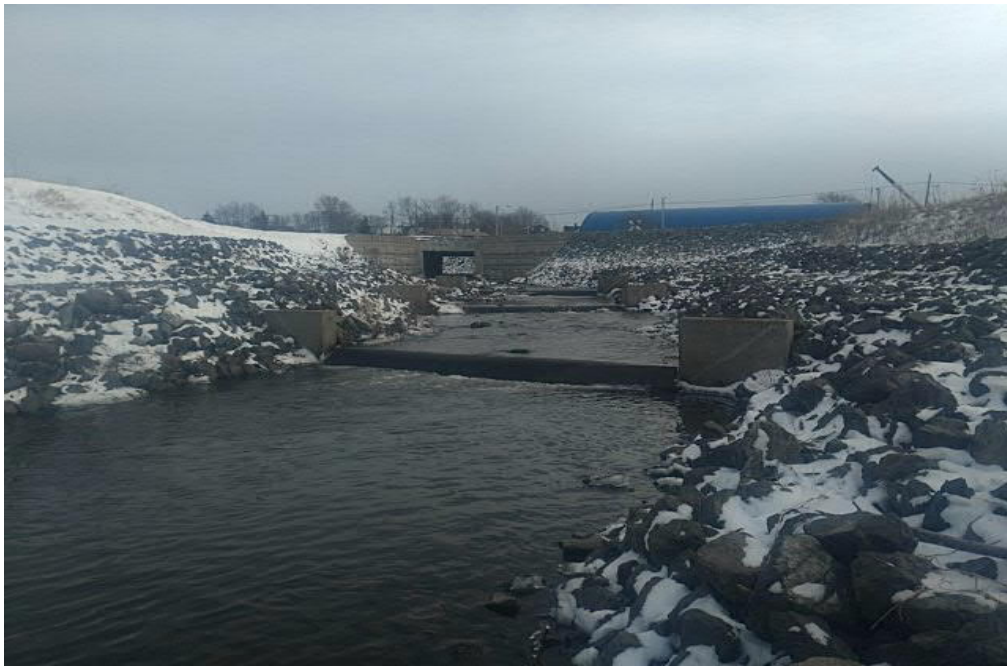
Photo No. 14: View of COB-6-SW looking northeast.
