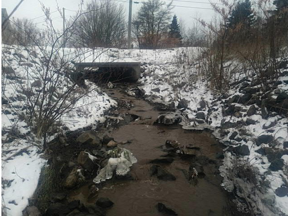
Photo No. 3: View of NRC-1-SW looking north.
