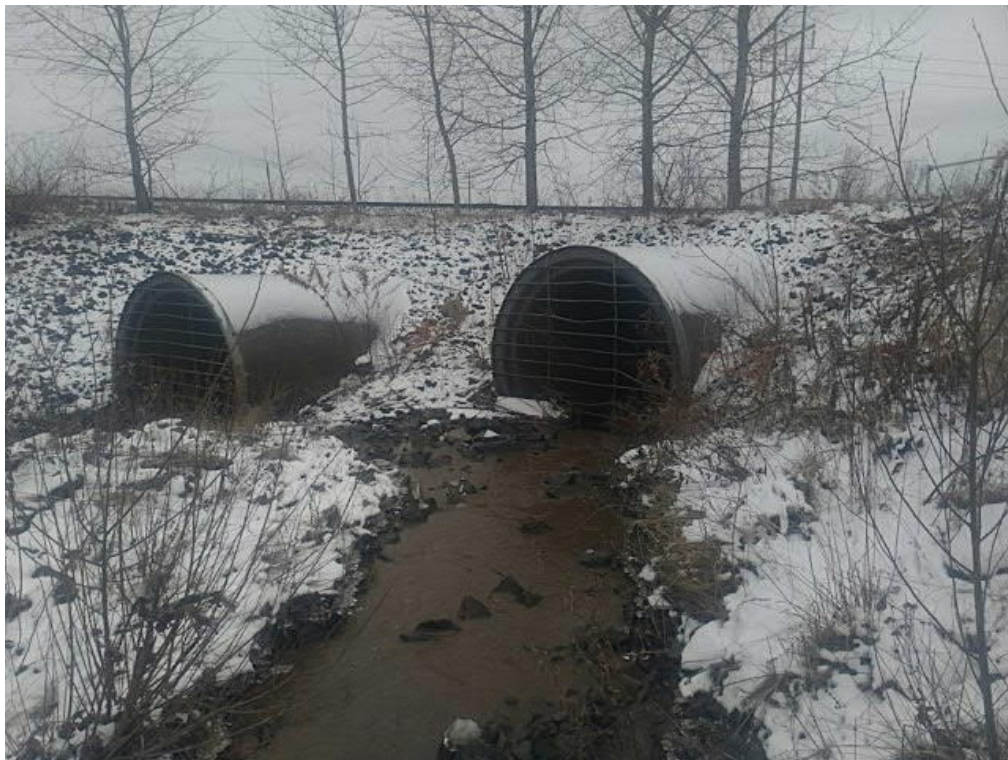
Photo No. 4: View of NRC-1-SW looking southeast.
