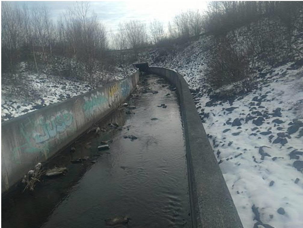
Photo No. 6: View of SRC-1-SW looking east.
