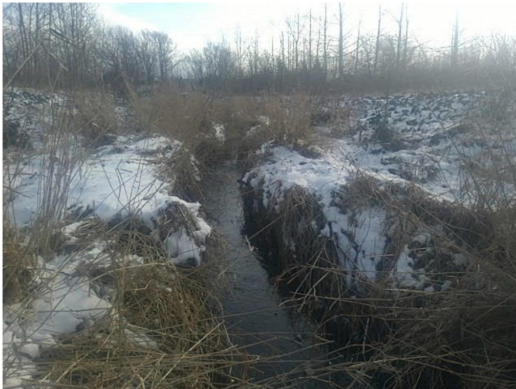
Photo No. 2: View of CB-SW looking southeast.
