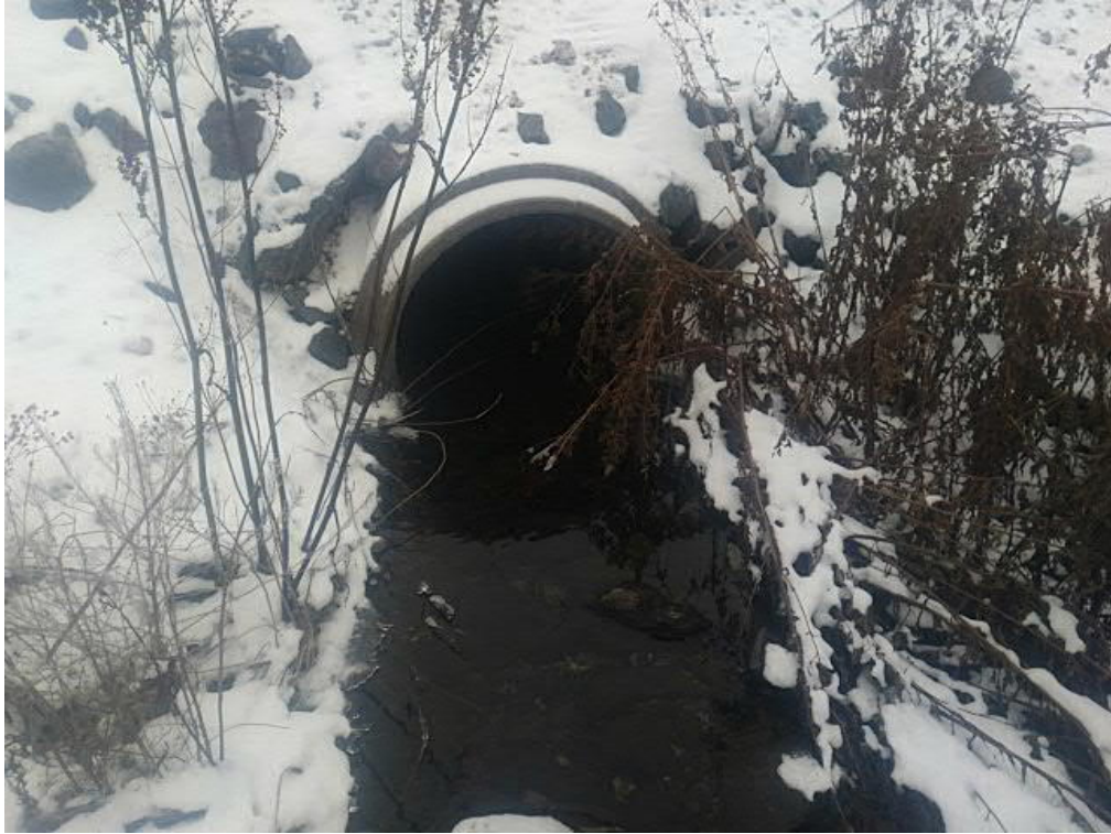
Photo No. 7: View northeast of COB-A-SW, looking northeast.
