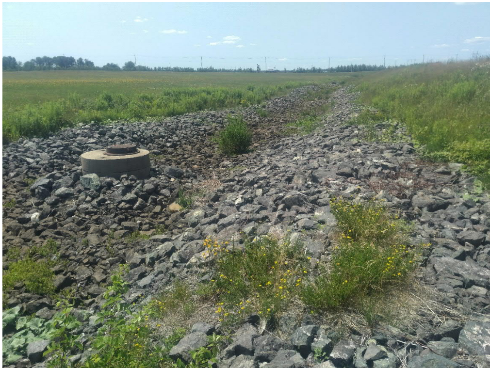
Photo No. 8: View of COB-A-SW looking west.
