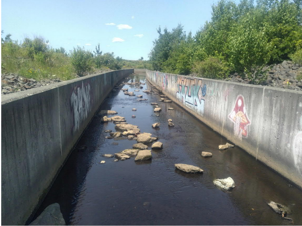
Photo No. 5: View of SRC-1-SW looking northwest.
