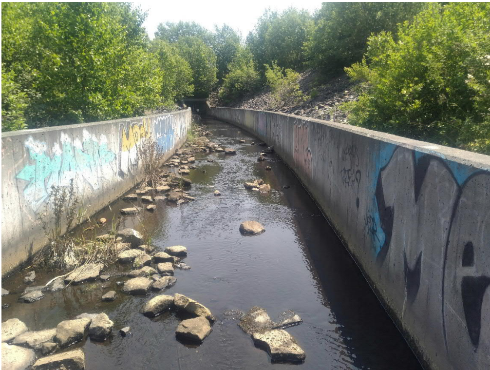
Photo No. 6: View of SRC-1-SW looking east.
