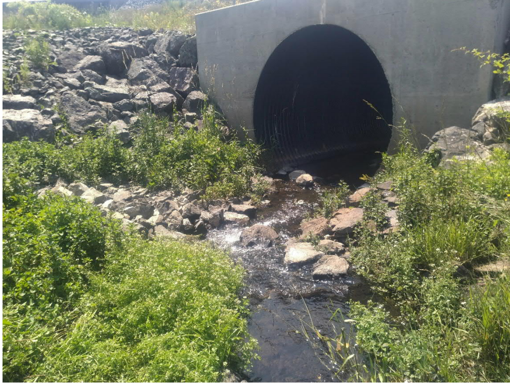
Photo No. 11: View of COB-4-SW looking west.
