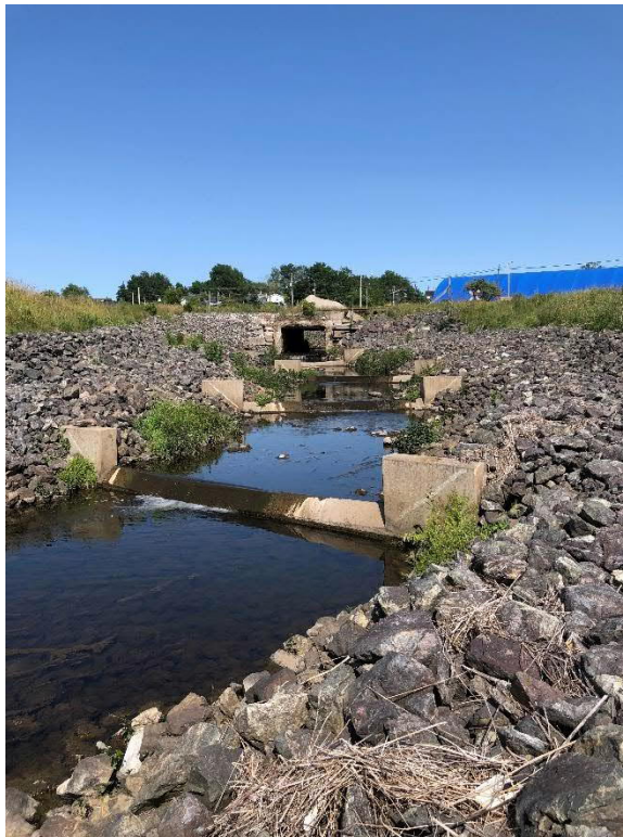
Photo No. 14: View of COB-6-SW looking northeast.
