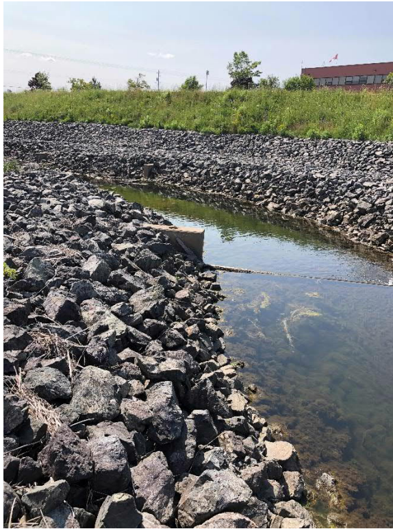
Photo No. 13: View of COB-6-SW looking west.
