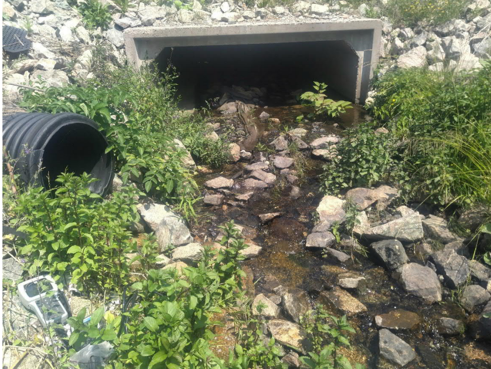
Photo No. 3: View of NRC-1-SW looking north.
