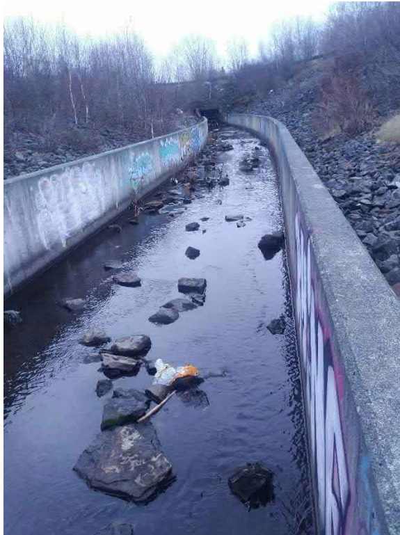
Photo No. 6: View of SRC-1-SW looking east.
