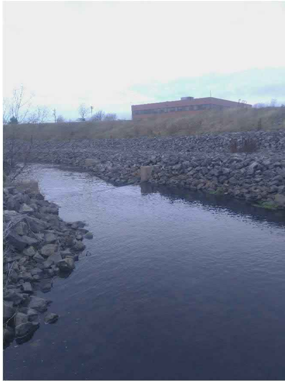
Photo No. 13: View of COB-6-SW looking west.
