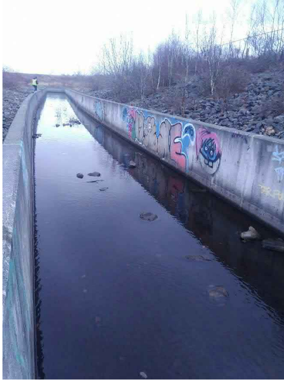
Photo No. 5: View of SRC-1-SW looking northwest.
