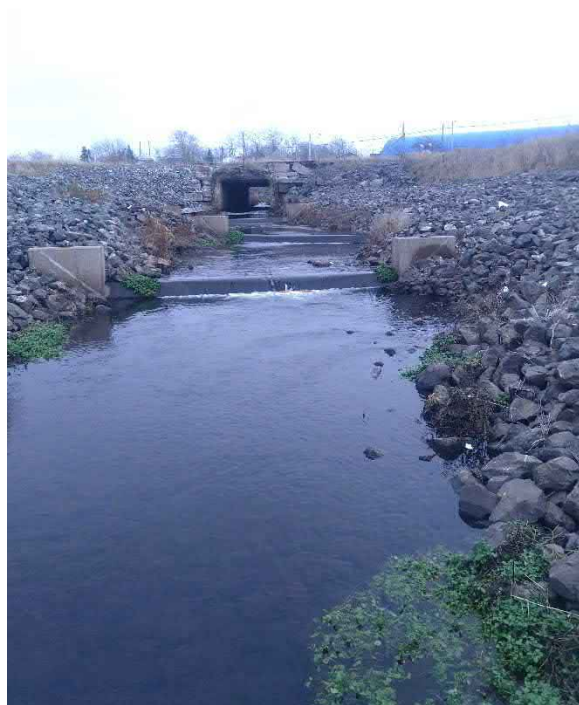
Photo No. 14: View of COB-6-SW looking northeast.
