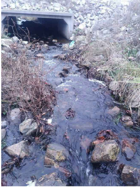
Photo No. 3: View of NRC-1-SW looking north.
