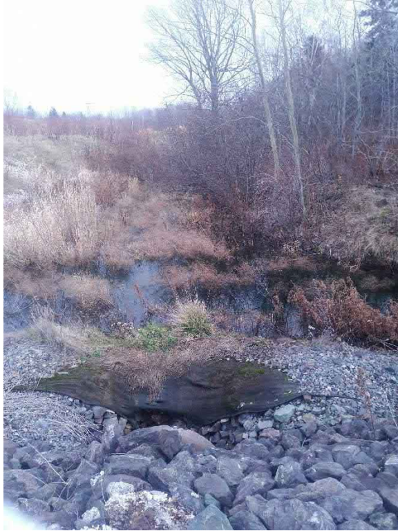
Photo No. 7: View northeast of COB-A-SW, looking northeast.
