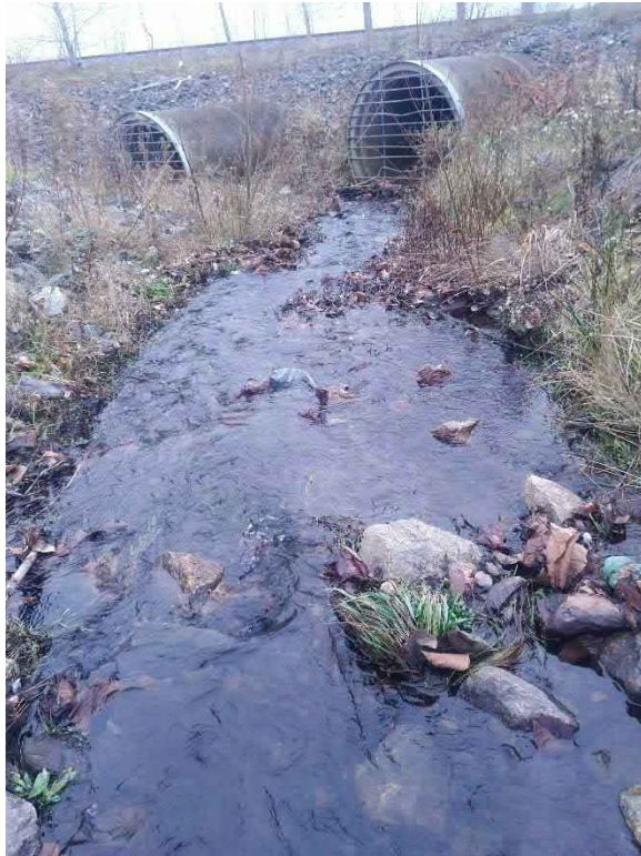
Photo No. 4: View of NRC-1-SW looking southeast.
