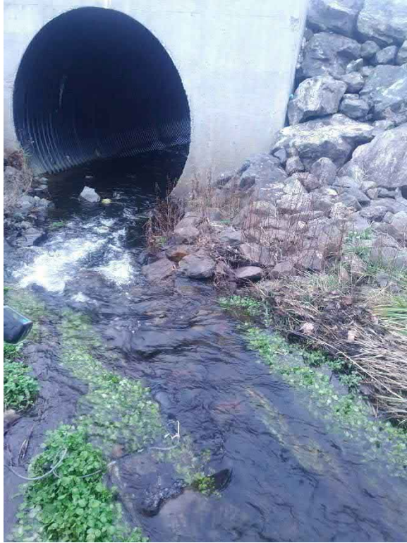
Photo No. 11: View of COB-4-SW looking west.
