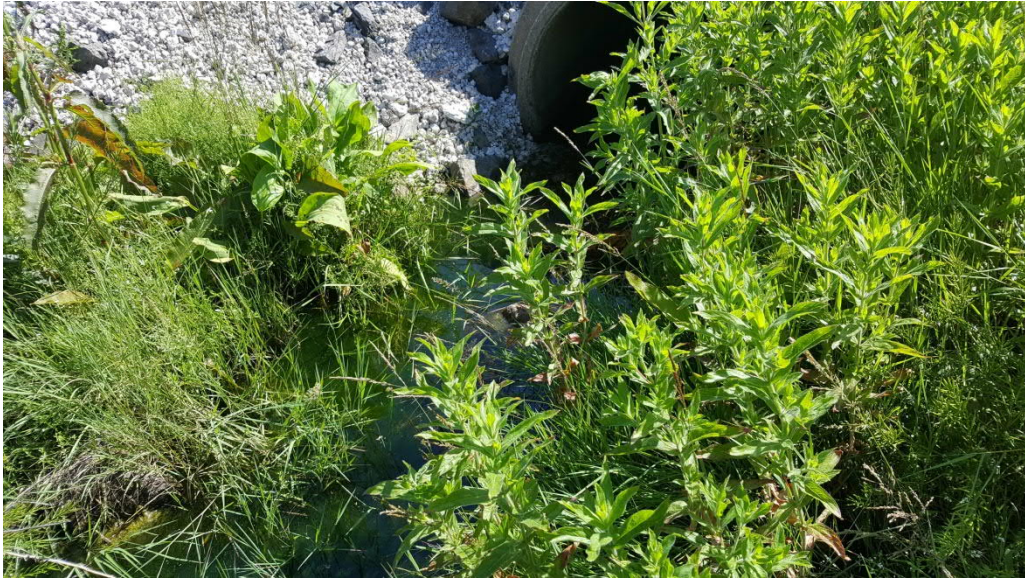
PHOTO No. 7: View of COB-A-SW looking northeast.
