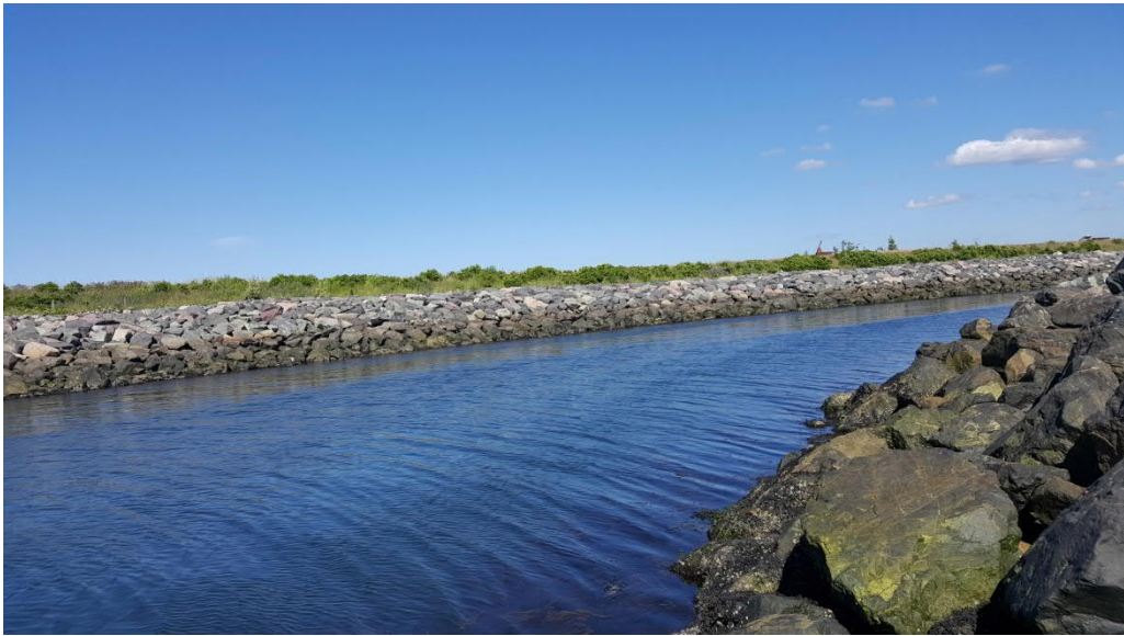
PHOTO No. 20: View of BP-1-SW looking southeast.
