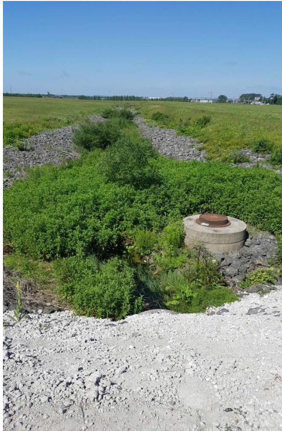
PHOTO No. 8: Overview of COB-A-SW looking west.
