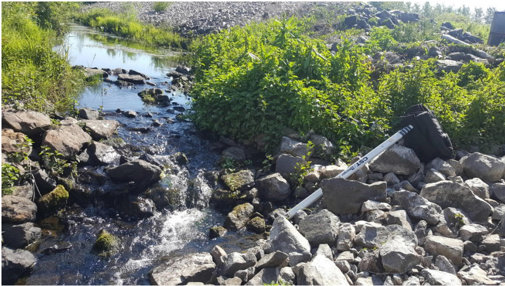
PHOTO No. 12: View of COB-4-SW looking northeast.
