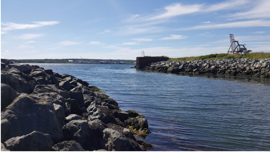
PHOTO No. 19: View of BP-1-SW looking northwest.
