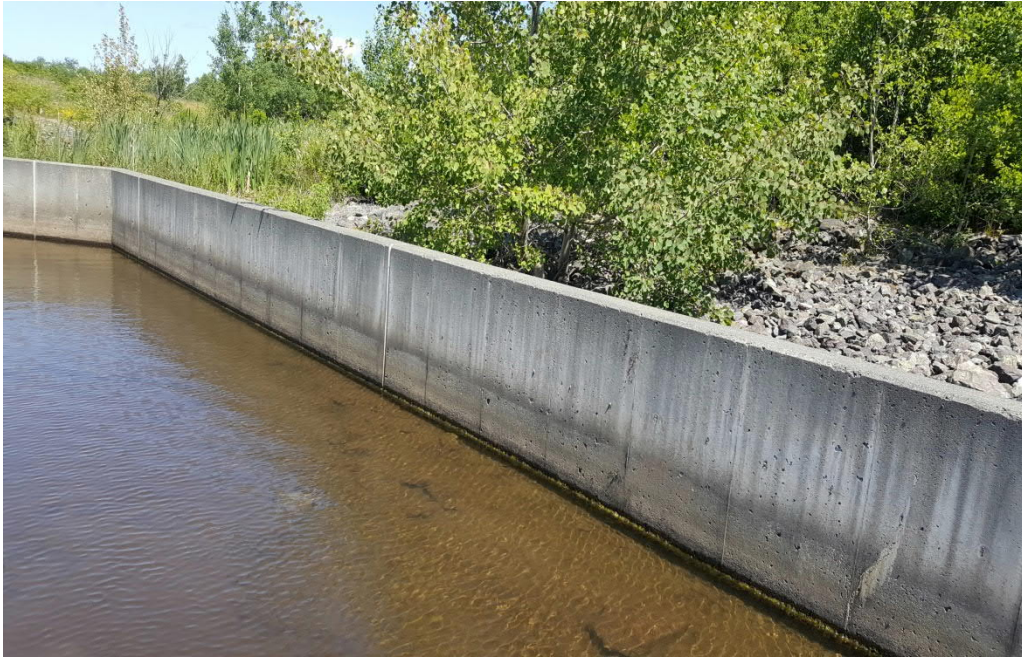
PHOTO No. 5: View of SRC-1-SW looking northwest.
