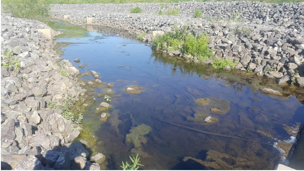
PHOTO No. 13: View of COB-6-SW looking west.
