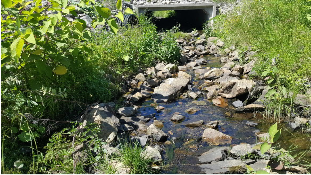
PHOTO No. 3: View of NRC-1-SW looking north.
