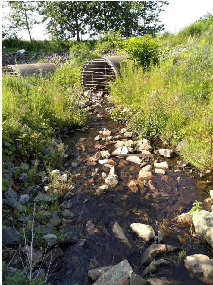
PHOTO No. 4: View of NRC-1-SW looking southeast.
