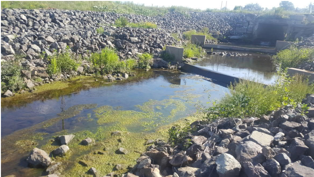
PHOTO No. 14: View of COB-6-SW looking northeast.
