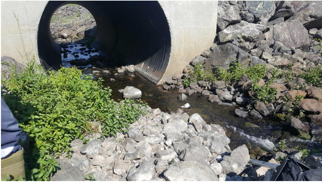
PHOTO No. 11: View of COB-4-SW looking northeast.
