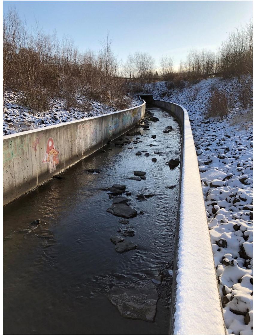
PHOTO 5: View of SRC-1-SW looking northeast.
