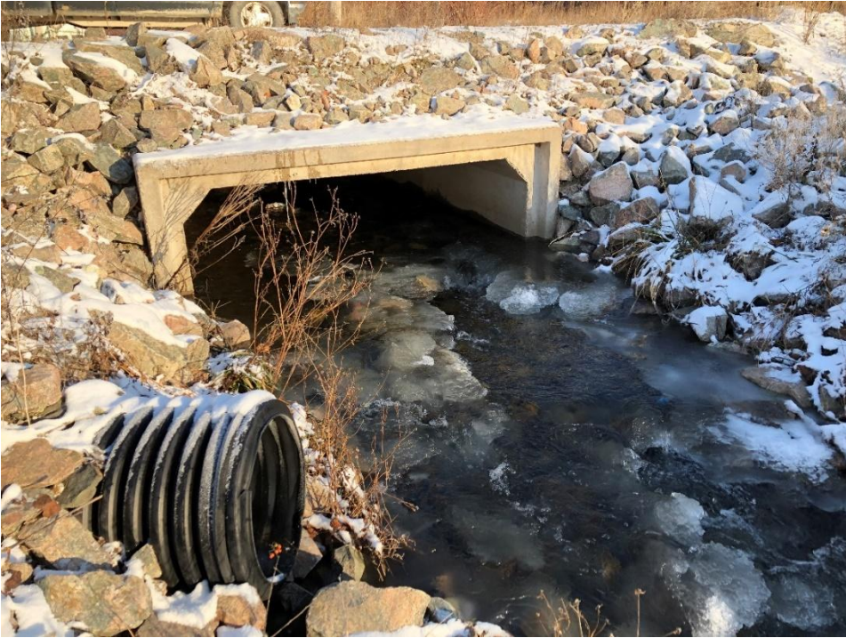
PHOTO 2: View of NRC-1-SW looking north.
