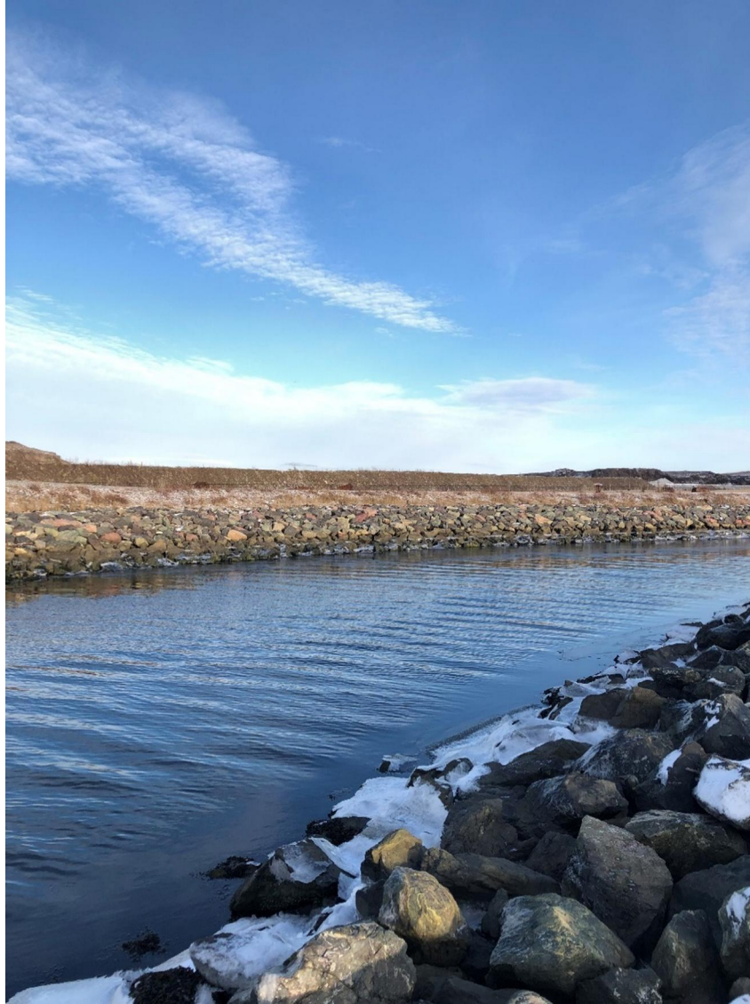
PHOTO 18: View of BP-1-SW looking east.
