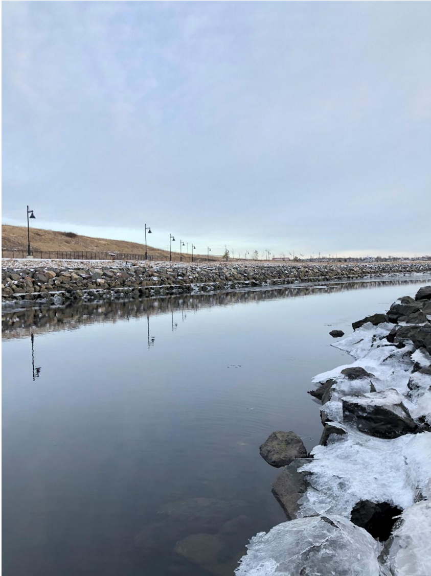
PHOTO 16: View of NARROWS looking southeast.
