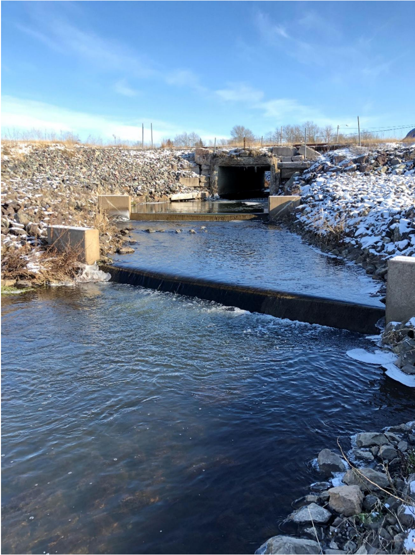
PHOTO 12: Upstream view from COB-6-SW looking northeast.
