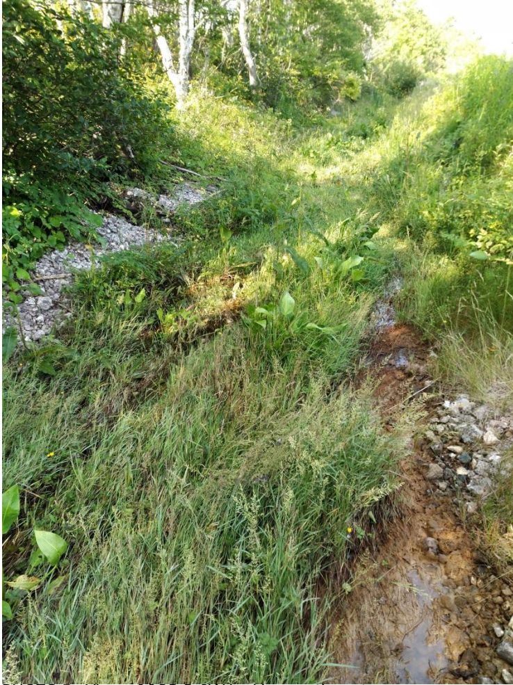
PHOTO 5: View of COB-B-SW looking southwest.
