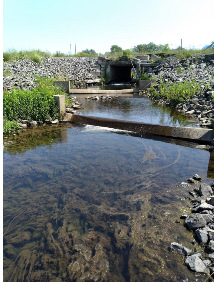
PHOTO 8: View of COB-6-SW looking northeast.
