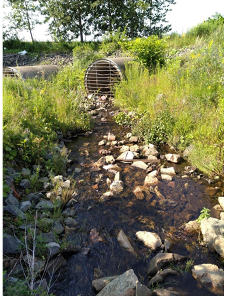
PHOTO 2: View from NRC-1-SW looking southeast.
