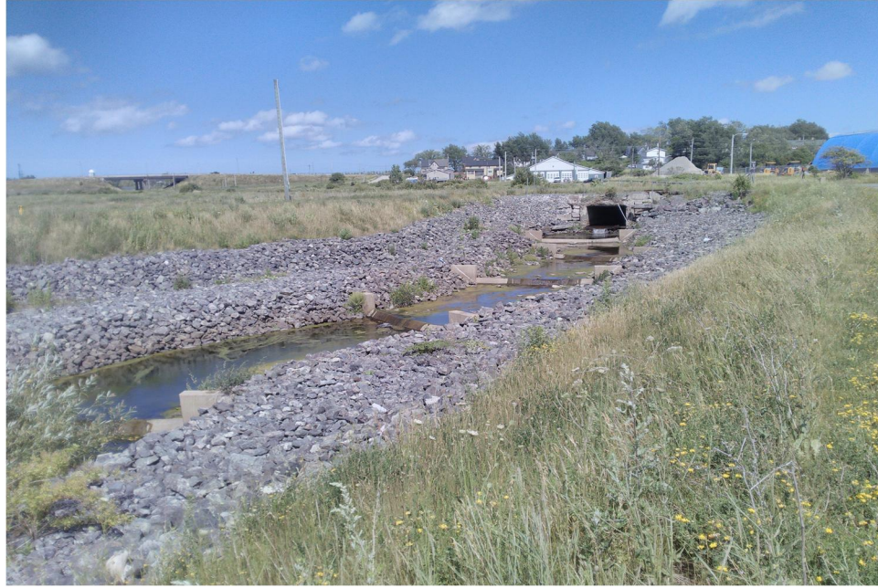
PHOTO 7: View of COB-6-SW looking northeast.
