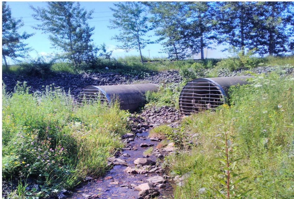
PHOTO 2: View looking from NRC-1-SW to the southeast.
