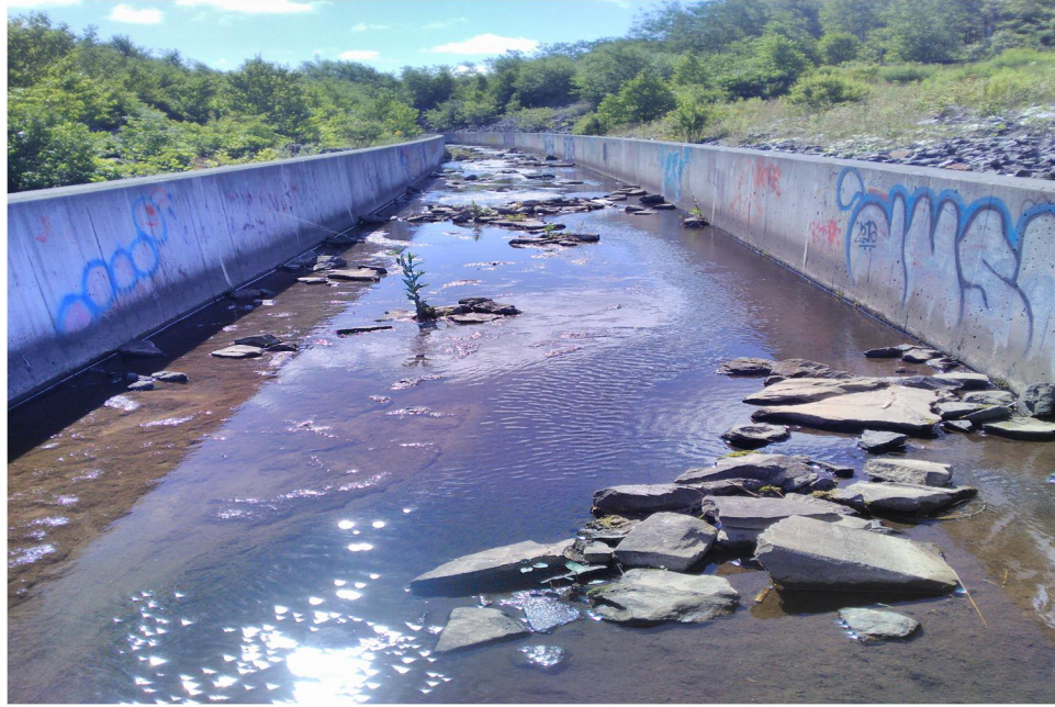
PHOTO 3: View of SRC-1-SW looking northeast.
