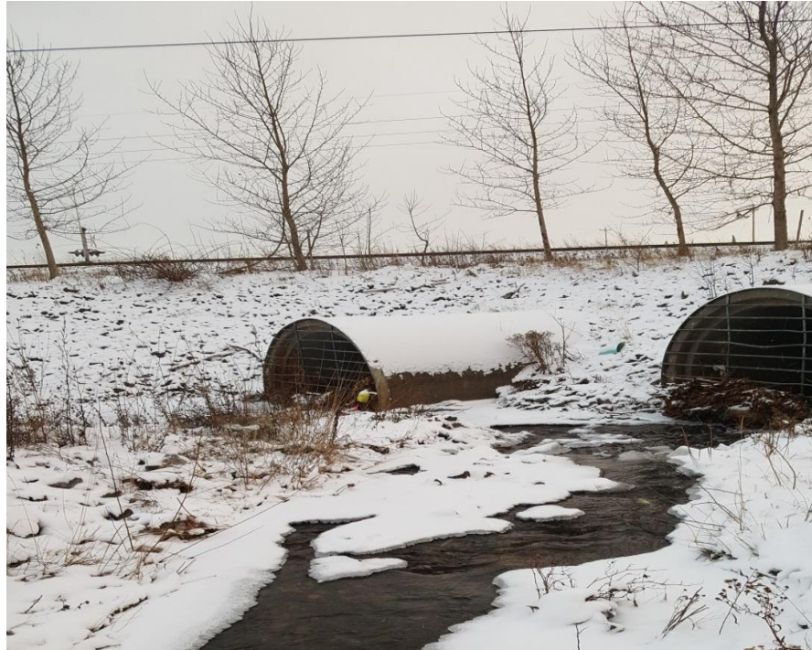
PHOTO 2: View looking from NRC-1-SW to the southeast.
