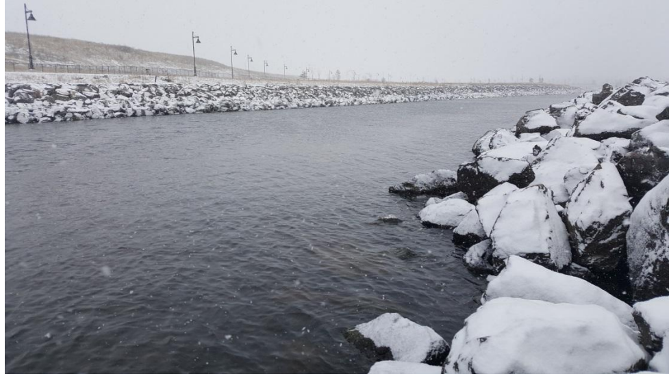
PHOTO 11: View of BP-1-SW looking southeast.
