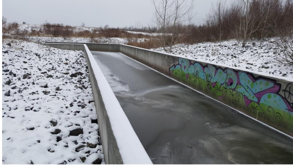
PHOTO 3: View of SRC-1-SW looking southwest.
