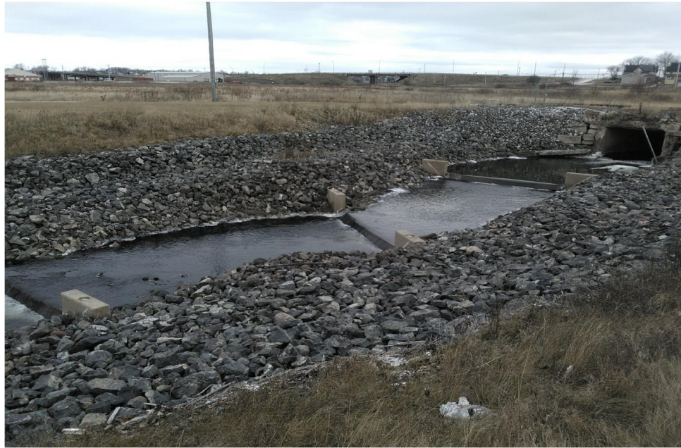
PHOTO 7: View of COB-6-SW looking northeast.
