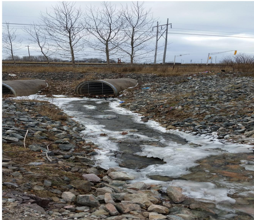
PHOTO 2: View looking from NRC-1-SW to the southeast.
