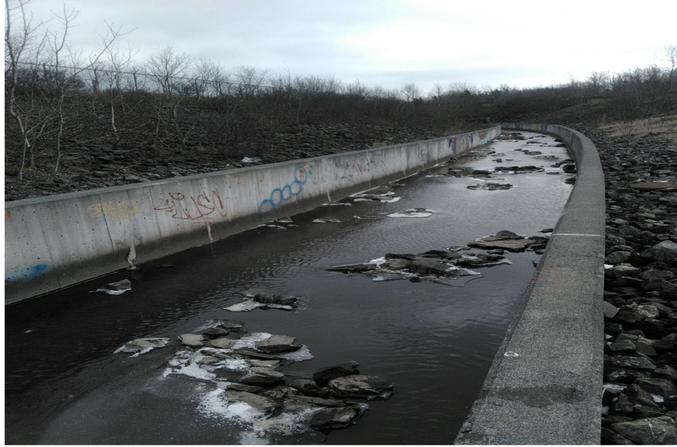
PHOTO 3: View of SRC-1-SW looking northeast.
