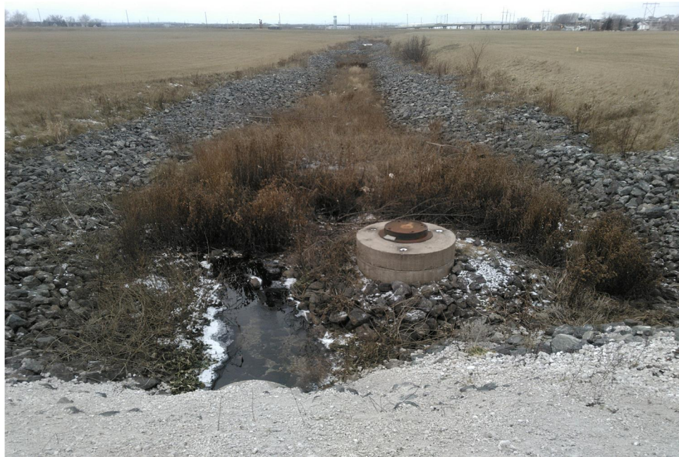
PHOTO 4: View of COB-A-SW looking west.
