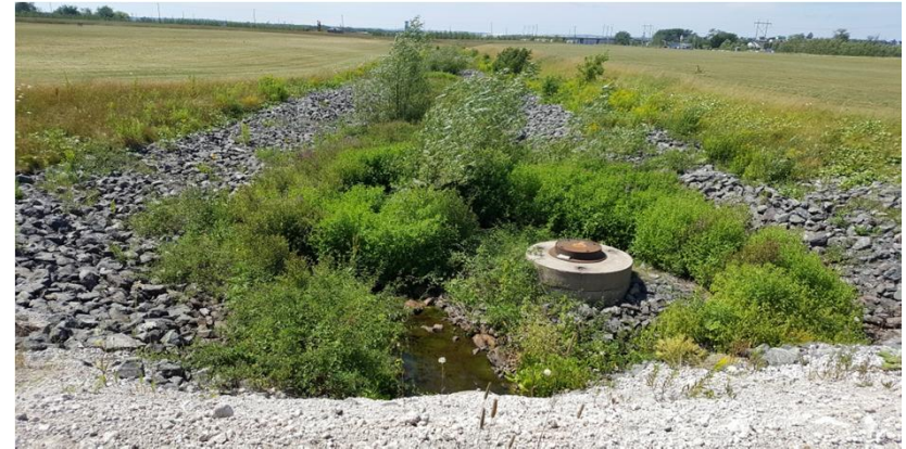
PHOTO 4: View of COB-A-SW looking west.
