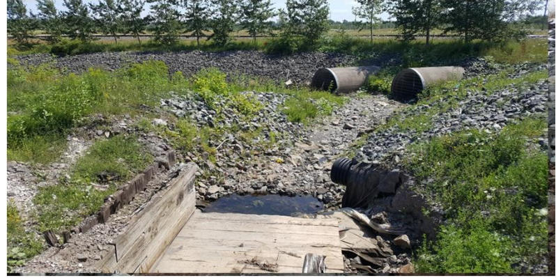
PHOTO 2: View of NRC-1-SW looking southeast.
