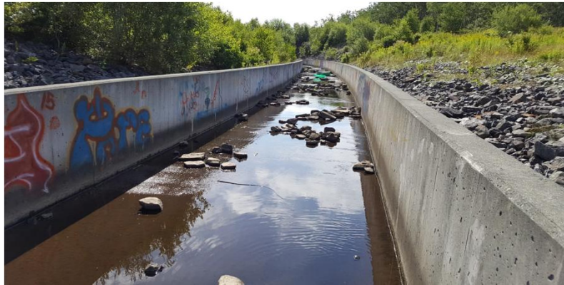
PHOTO 3: View of SRC-1-SW looking northeast.
