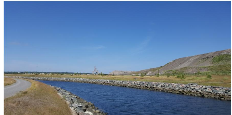
PHOTO 10: View of NARROWS looking west.
