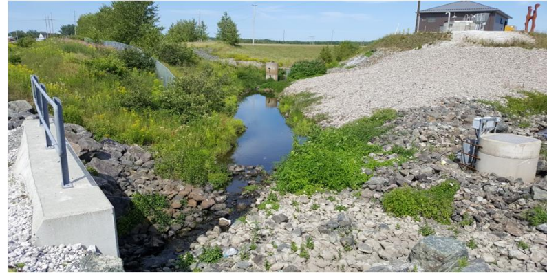
PHOTO 6: View of COB-4-SW looking northeast.
