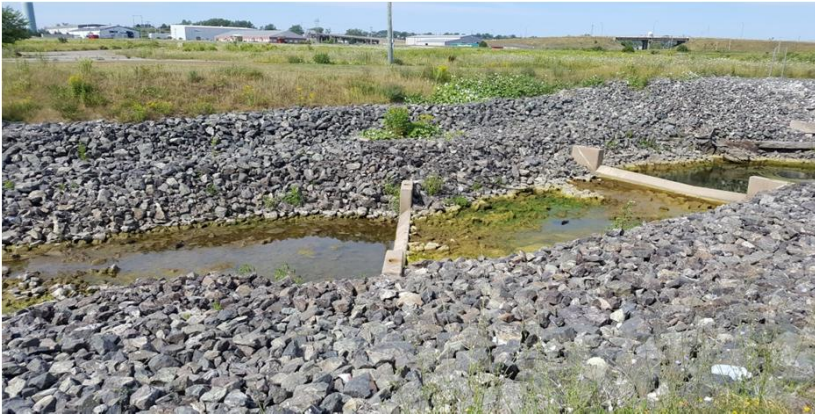
PHOTO 7: View of COB-6-SW looking northwest.
