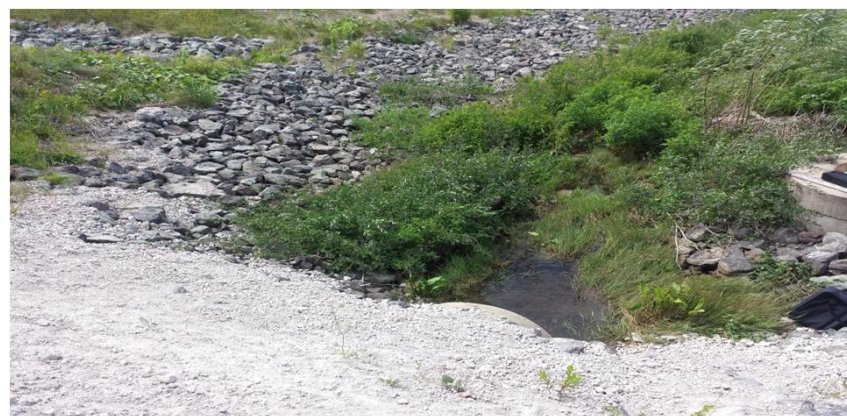
PHOTO 4: View of COB-A-SW looking northwest. Stagnant water visible.
