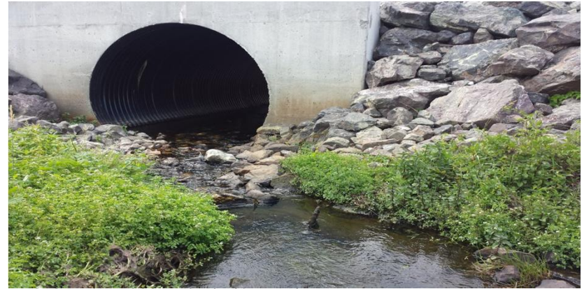
PHOTO 6: View of COB-4-SW looking northwest.
