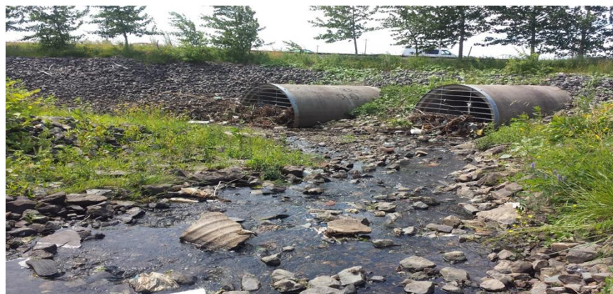
PHOTO 2: View of NRC-1-SW looking southeast.
