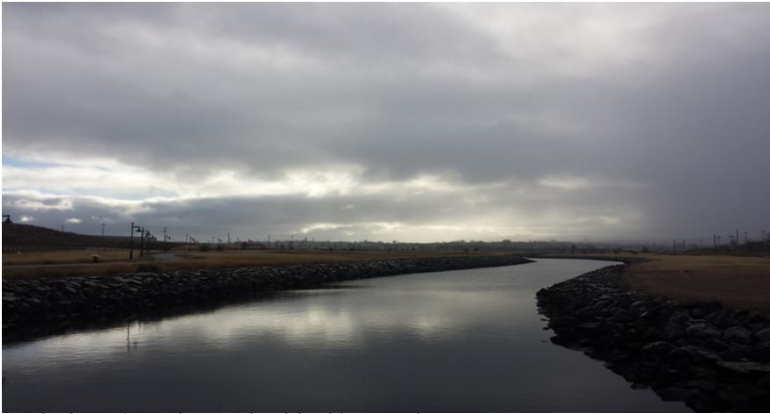
PHOTO 9: View of NARROWS looking southeast.
