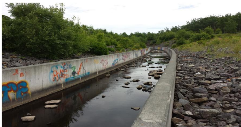
PHOTO 3: View of SRC-1-SW looking northeast.
