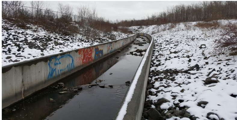
PHOTO 3: View of SRC-1-SW looking northeast.
