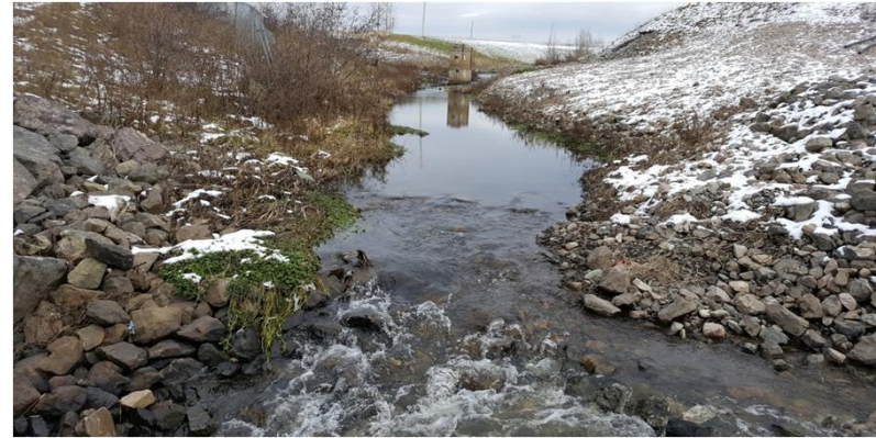
PHOTO 6: View of COB-4-SW looking northeast.
