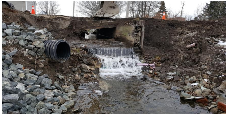
PHOTO 11: View of NRC-1-SW looking northwest to a culvert replacement that was taking place immediately up-gradient of the surface water station.
