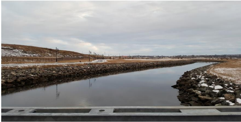
PHOTO 9: View of NARROWS looking southeast.
