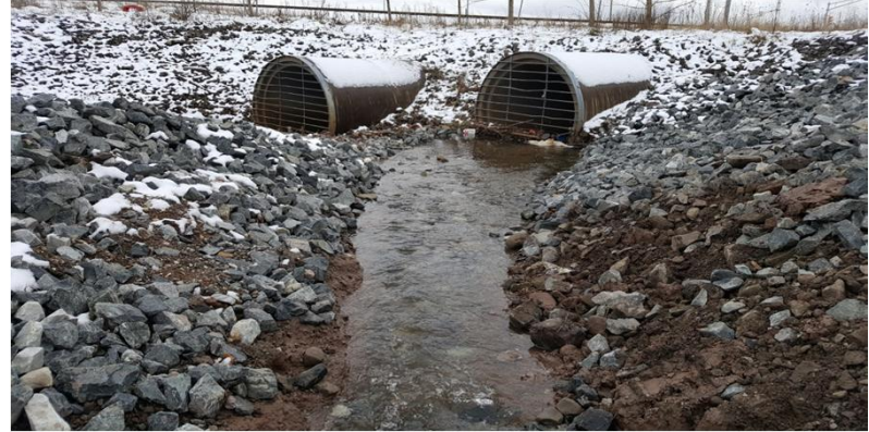
PHOTO 2: View of NRC-1-SW looking southeast.
