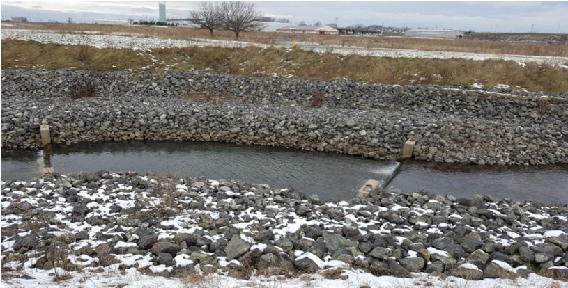
PHOTO 7: View of COB-6-SW looking northwest.
