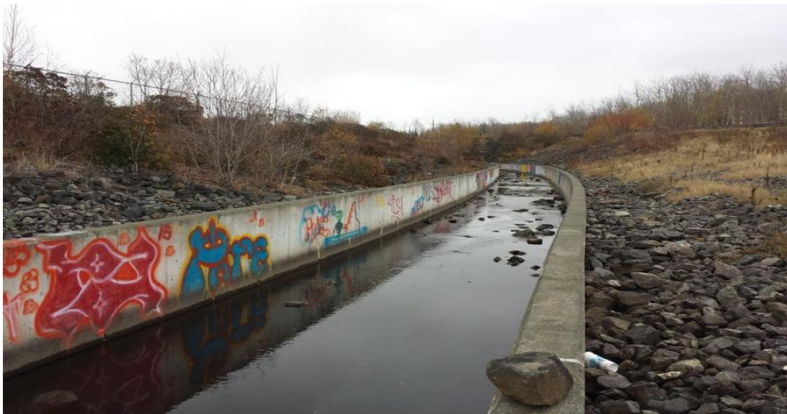
PHOTO 3: View of SRC-1-SW looking northeast.
