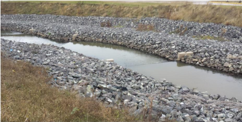
PHOTO 7: View of COB-6-SW looking northwest.
